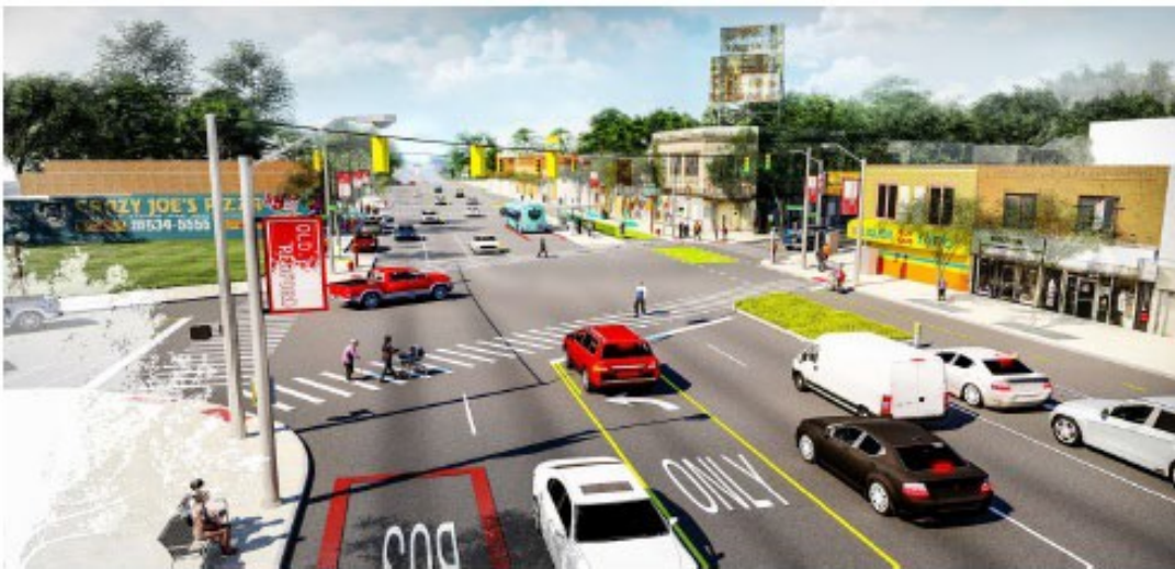
Grand River Streetscape Project, 2020 – Detroit Department of Public Works
