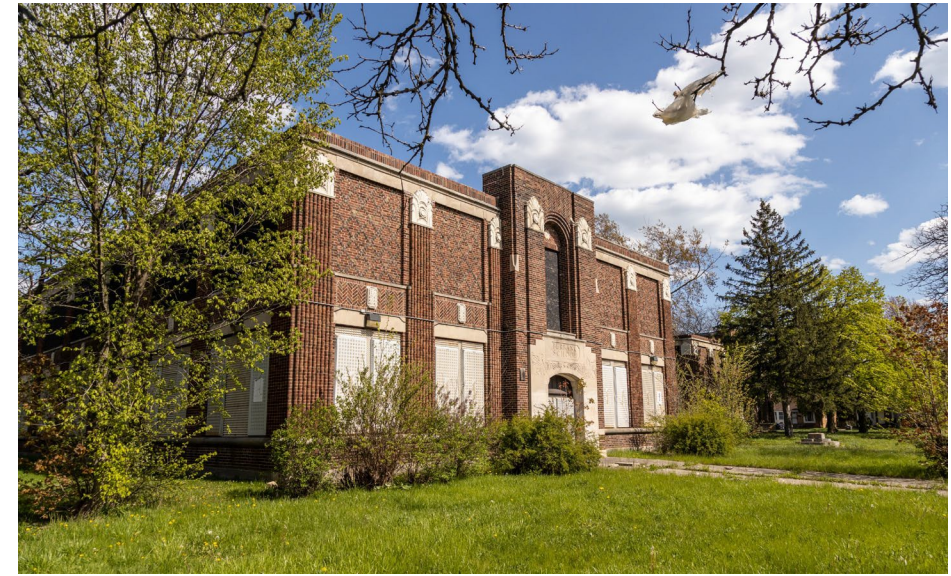
Former Burbank Elementary
