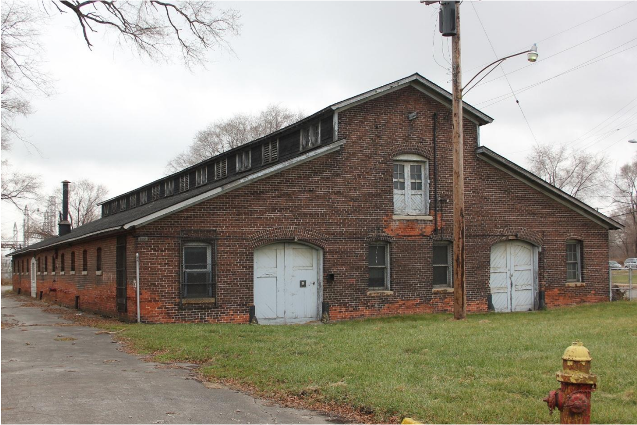
Front (northeast) facade, February 2017
