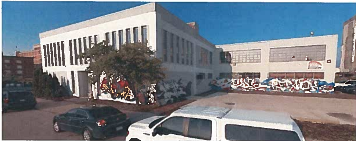
Two views of the current condition of the building at 1401 Vermont
