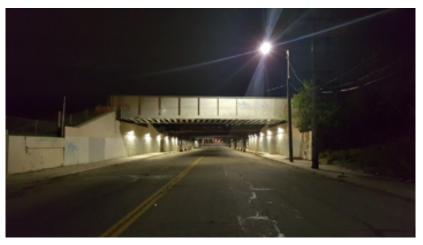
This viaduct, one of several crossing Junction Street, is a good model for improvements to other viaducts: well-lit sideway and roadway area, stable and clean foundation walls, functioning drainage. Most other viaducts have multiple support piers between their abutments, requiring additional light fixtures to achieve consistent lighting levels.
