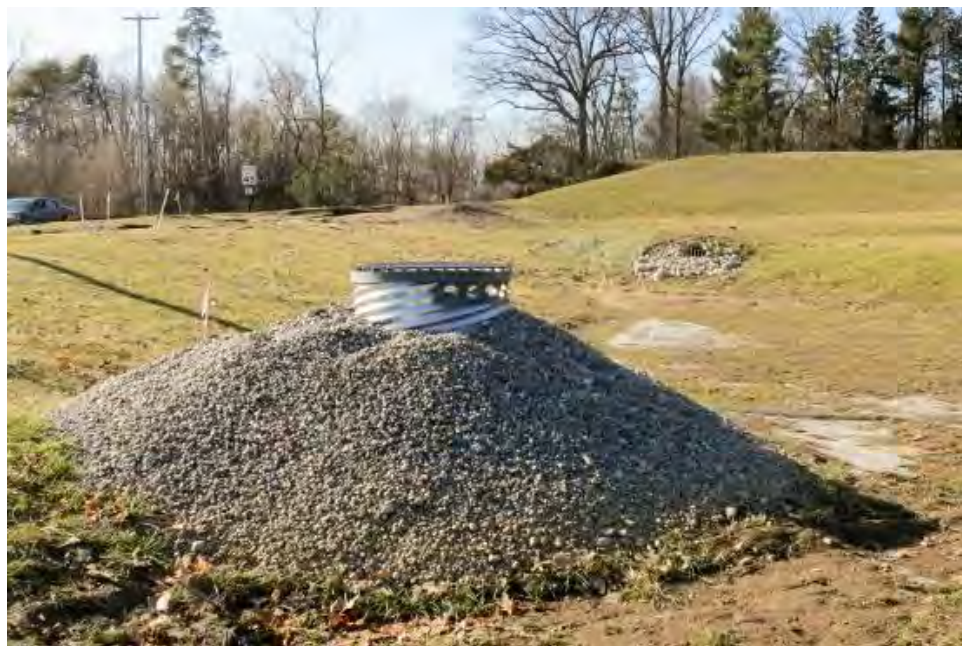
Figure 7-14 Typical Riser Pipe with Stone Jacket
