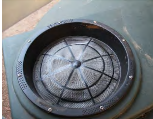
Figure 10-5 Filter at the Inlet on a Cistern
