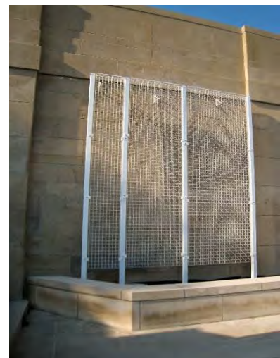
Figure 12-15 Green façade wall-mounted trellis system
