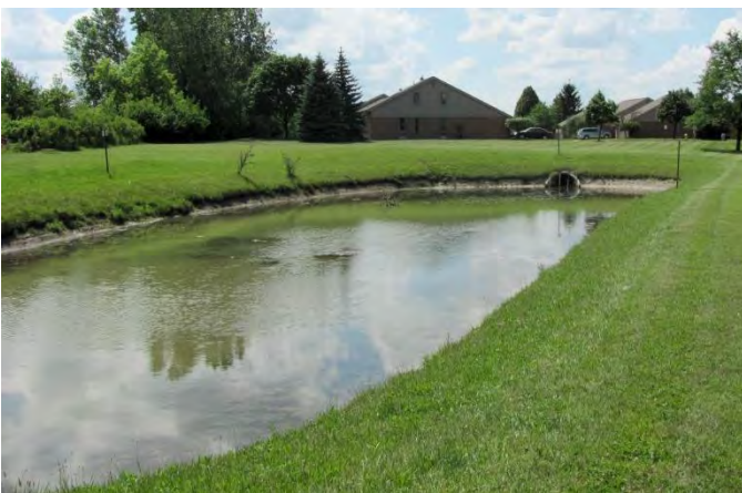
Figure 7-6 Detention with a Permanent Pool
