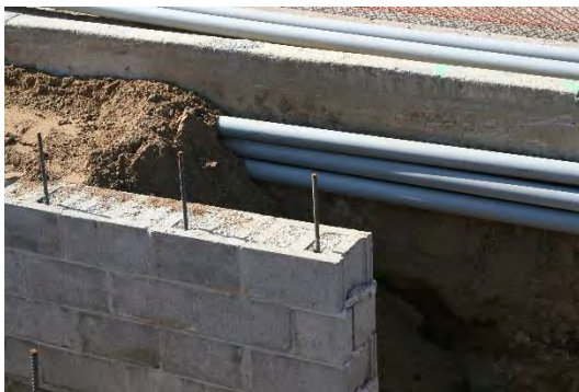
Figure 15-14 Example of electrical conduits in a tree box
