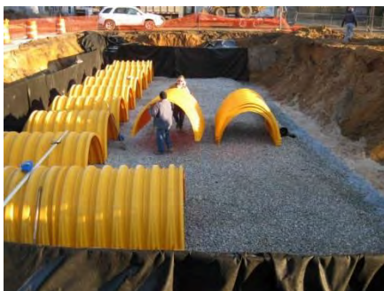
Figure 9-4 Infiltration Vault
