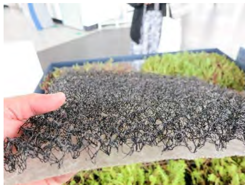
Figure 12-10 Living roof drainage layer
