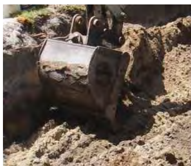
Figure 8-38 Scarifying soil with a toothed excavator bucket
