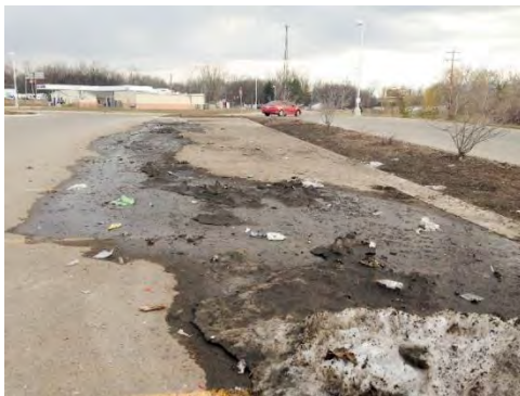
Figure 9-8 Typical trash and sediment left from melting snow piles
