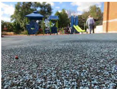
Figure 10-9 Example Rubber Overlay
