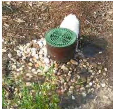
Figure 8-23 Upturned inlet
