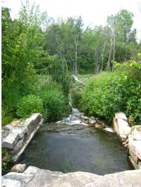
Figure 13-3 Stormwater Wetland Inlet
