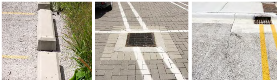
Pervious concrete parking; overflow conveyance to bioretention
