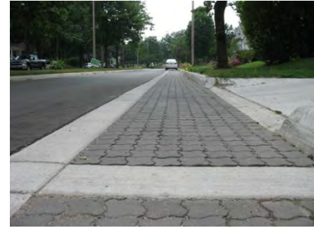
Figure 1-5 Permeable concrete pavers
