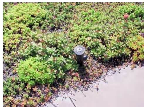
Figure 12-21 Overhead spray irrigation on vegetated roof
