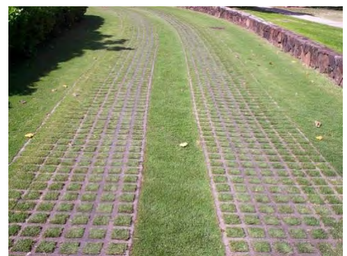
Figure 10-14 Permeable Access Road
