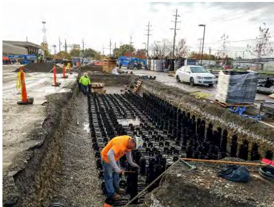
Figure 15-2 Installation of soil cells
