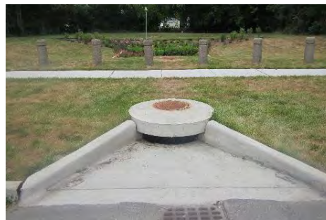
Figure 8-19 Curb cut bypassing CB
