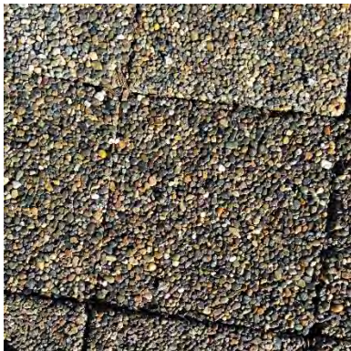
Figure 10-8 Example of Pervious Paver
