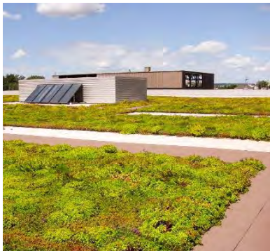
Figure 12-22 Concrete paver paths for maintenance access
