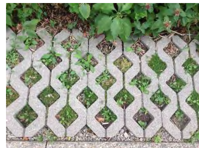
Figure 10-5 Example of Permeable Interlocking Concrete Pavers
