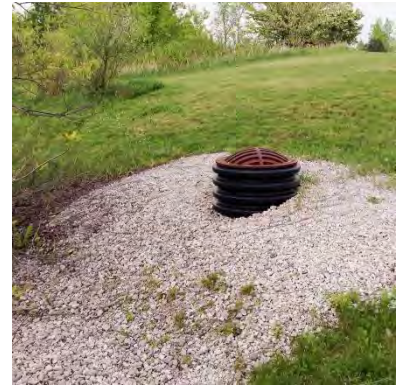
Figure 7-9 Aggregate Jacket Example
