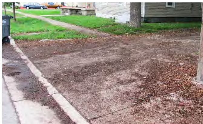
Figure 10-16 Permeable pavement with significant leaf litter
