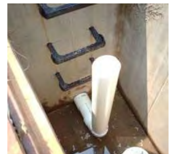
Figure 8-28 Upturned underdrain with capped tee connection
