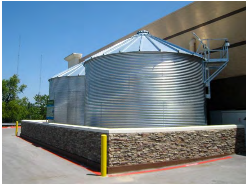
Figure 11-1 Cistern Example Used for Irrigation
