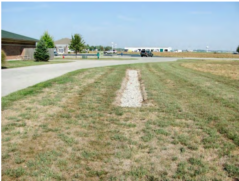
Figure 9-1 Infiltration trench installed adjacent to drive lane
