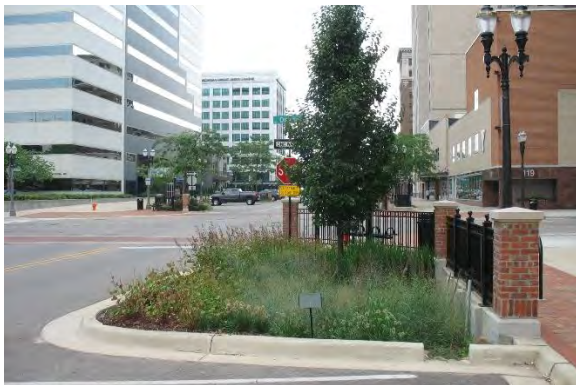
Figure 8-10 CBD Curb Extension Bioretention
