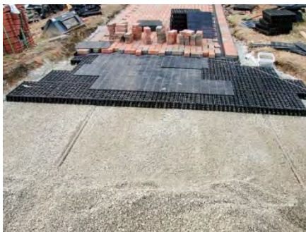
Figure 9-3 Infiltration Bed
