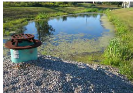
Figure 1-3 Retention basin with outlet riser
