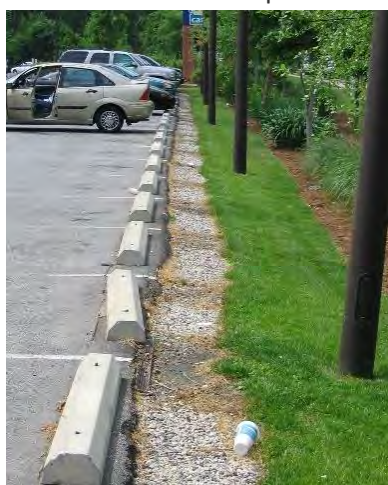
Figure 8-24 Vegetated filter strip leading to bioretention
