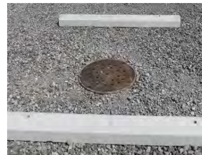
Figure 8-26 Permeable aggregate parking lot outlet structure
