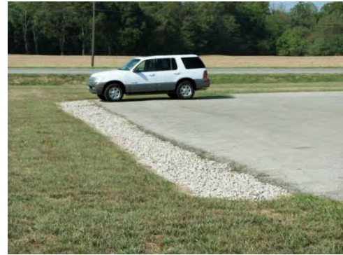
Figure 9-5 Infiltration Trench
