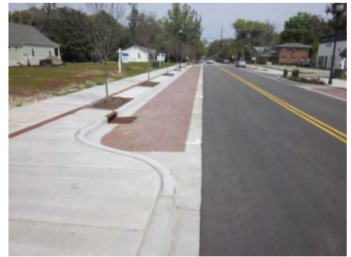
Figure 10-11 Permeable Parking Lane
