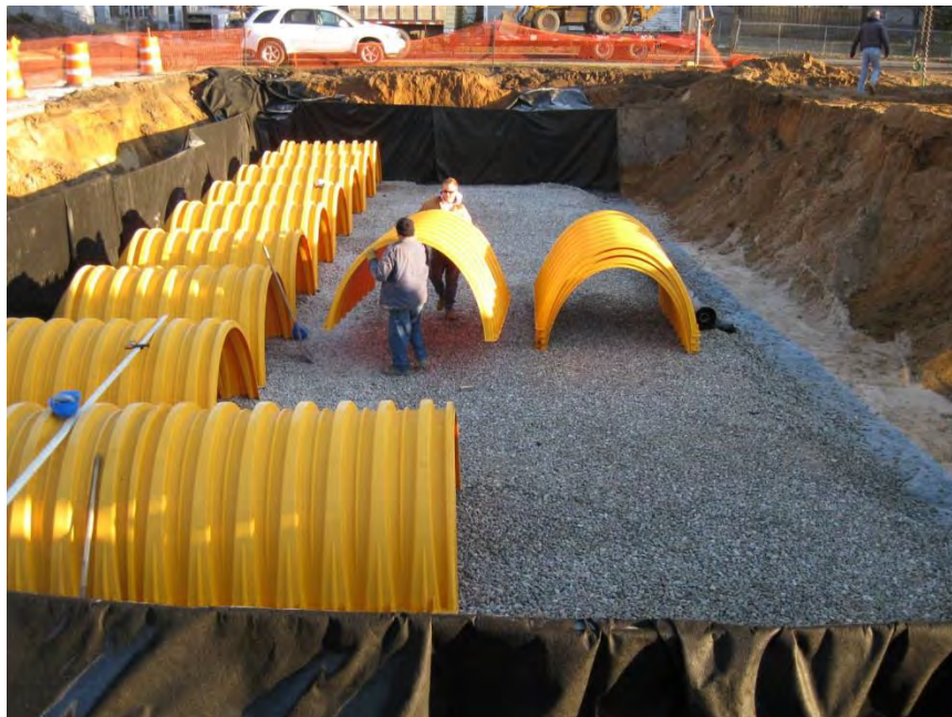
Figure 7-11 Subsurface Detention During Construction
