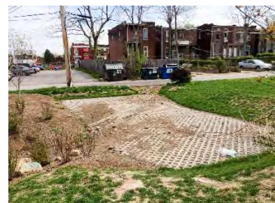
Figure 9-12 Sediment forebay
