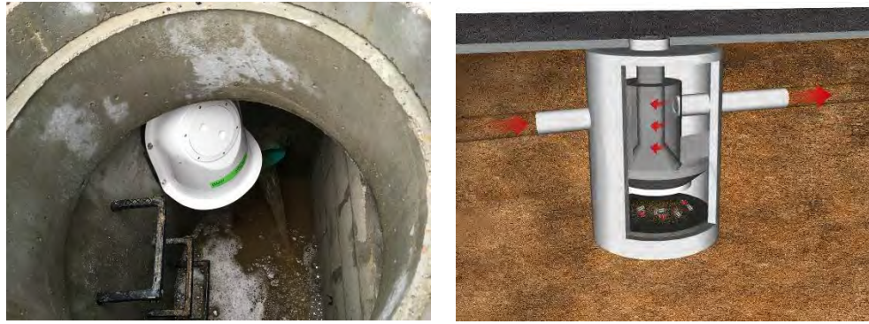
Figure 5-9 Gross Solids Removal Devices
