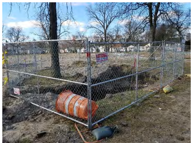
Figure 15-17 Tree protection removed for excavation
