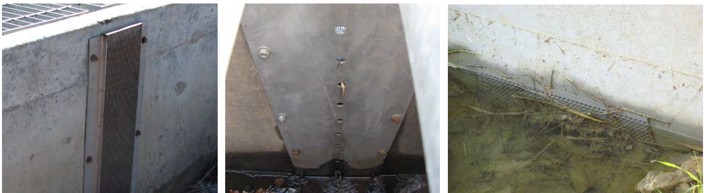
Specialty screen protecting orifice plate from clogging, outside (left); orifice plate, inside (center); clogged poorly designed screen (right)
