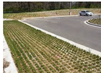
Figure 10-6 Example of Grid Pavement Systems
