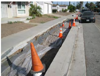
Figure 10-34 Protection of subgrade during construction
