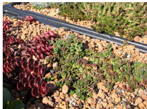
Figure 12-11 Typical composition of lightweight soil media for living roofs
