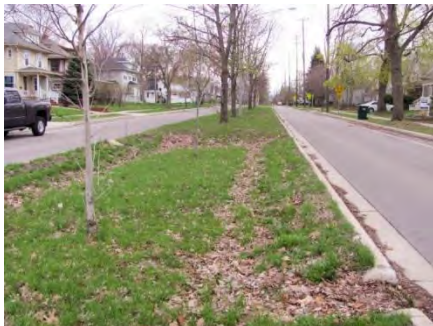
Figure 9-2 Infiltration Basin
