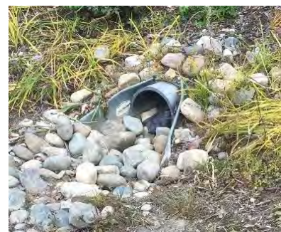
Figure 8-22 Piped inlet
