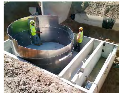
Figure 9-13 Installation of typical manufactured treatment device
