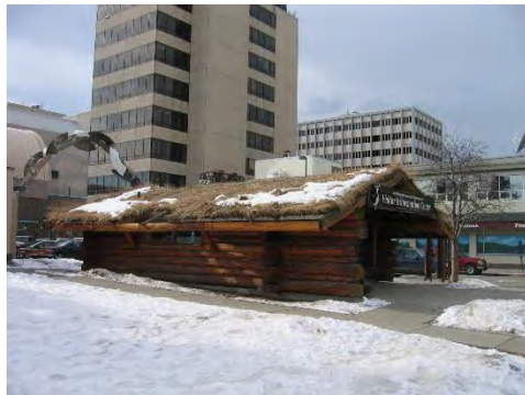
Figure 12-8 Sloped living roof installation in Alaska
