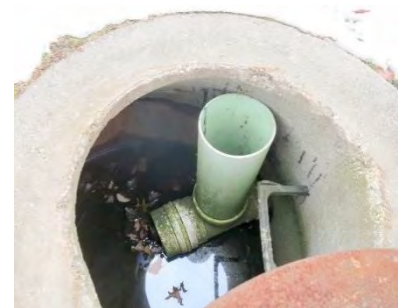
Figure 10-26 Upturned underdrain with a capped tee connection
