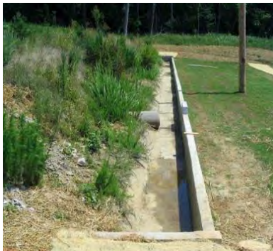
Figure 9-10 Typical level spreader
