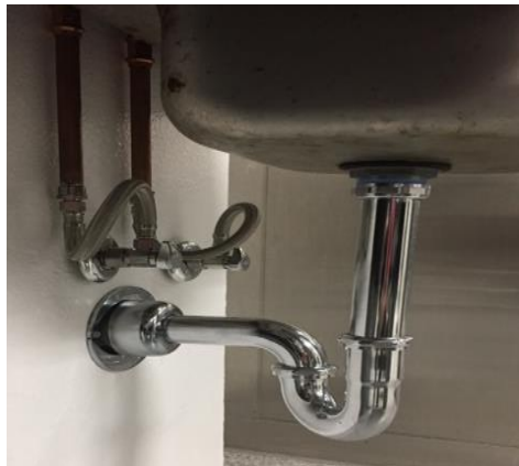
Direct connection- not permitted on equipment in which food, portable equipment or utensils are placed
