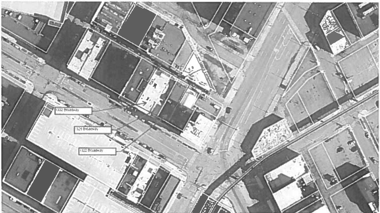
Site of the Broadway Lofts Development Project
