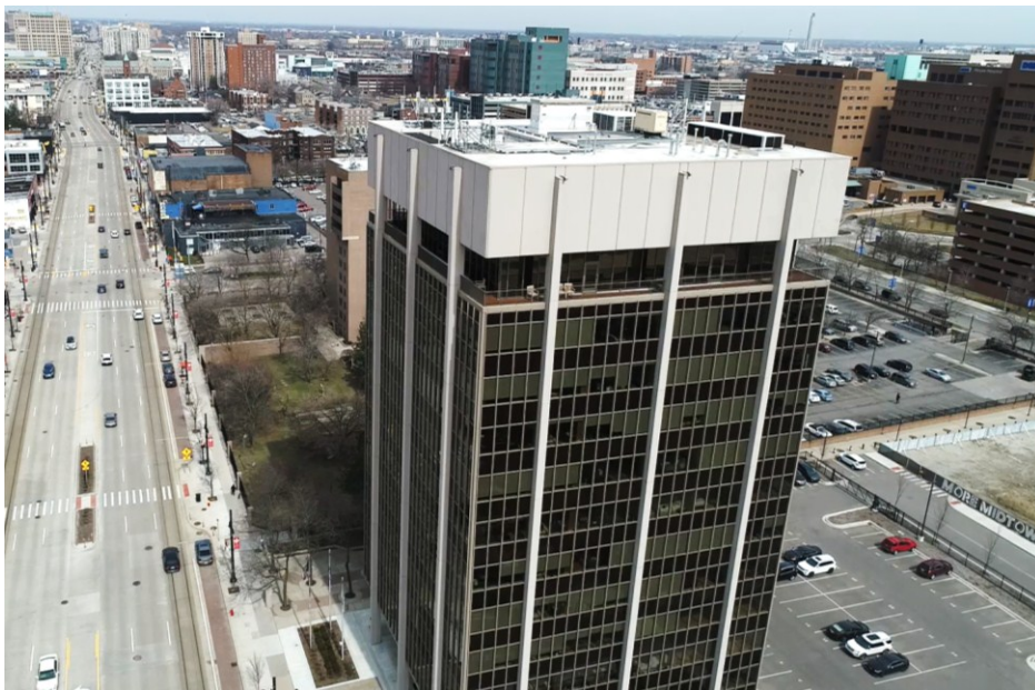
3800 Woodward, The Professional Plaza Tower ‘Hammer and Nail Building; existing.
