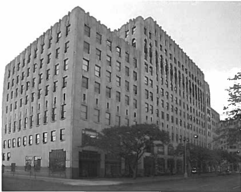
Albert Kahn Building
