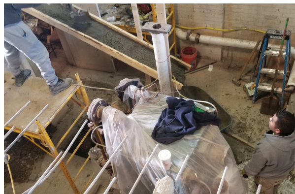
Pouring concrete for the new foundation at Engine 42.
