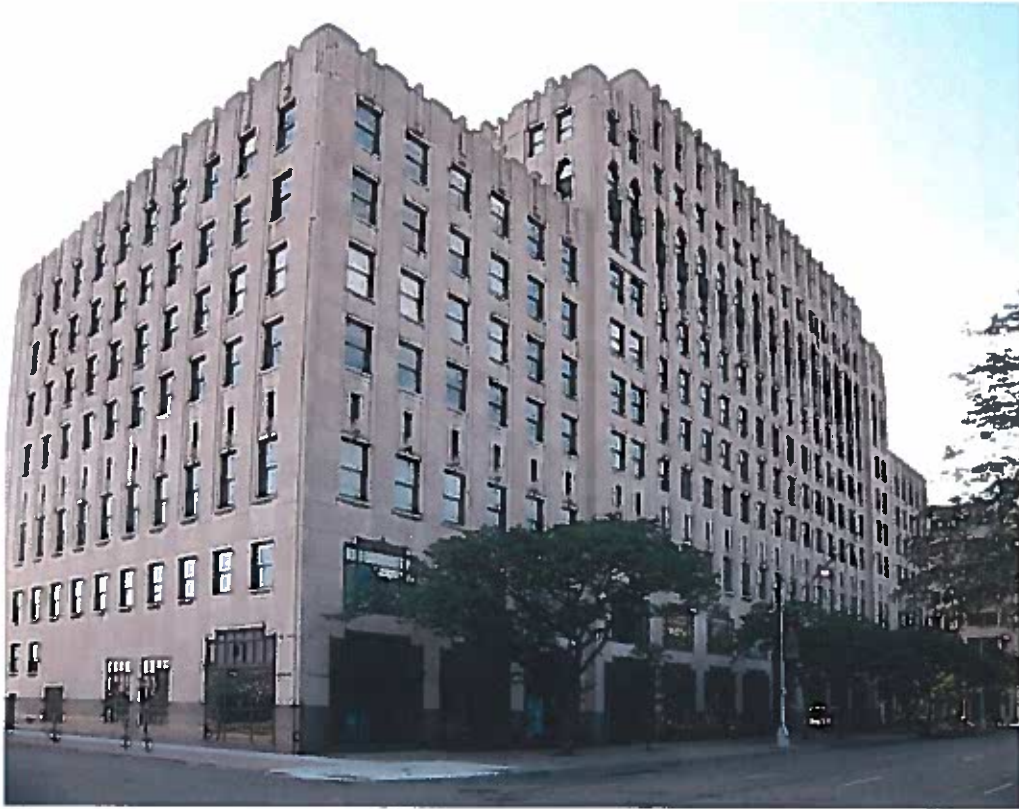
Albert Kahn Building
