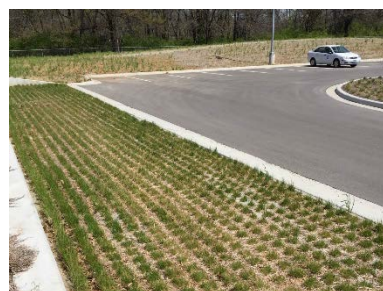
Figure 10-6 Example of Grid Pavement Systems
