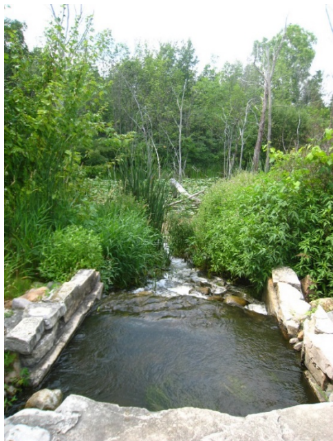
Figure 13-3 Stormwater Wetland Inlet
