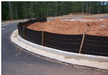
Silt fence at a construction site
