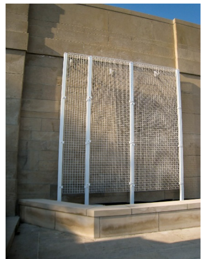
Figure 12-15 Green façade wall-mounted trellis system
