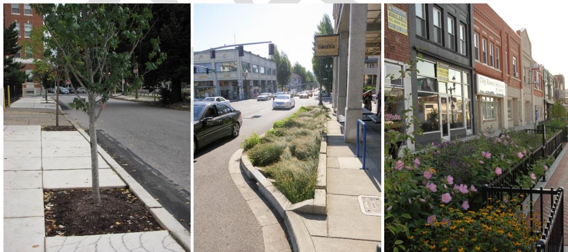
Three examples of green stormwater infrastructure practices in commercial district with similar benefits but different designs and costs. From left to right: tree based suspended pavement (Philadelphia PA), curb extension bioretention (Portland OR), and planter box (Lansing, MI).
