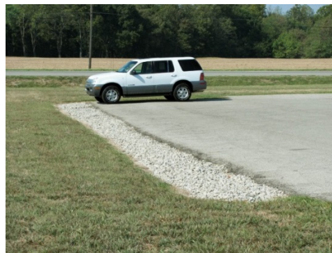
Figure 9-5 Infiltration Trench
