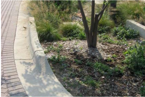
Figure 8-8 Parking Lot Bioretention
