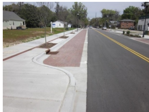
Figure 10-11 Permeable Parking Lane
