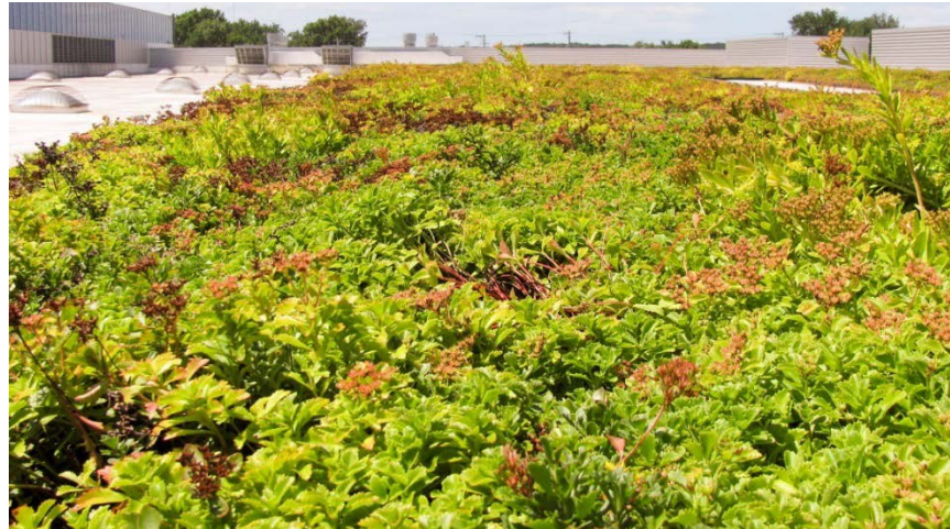
Figure 12-16 Typical low-growing living roof vegetation
