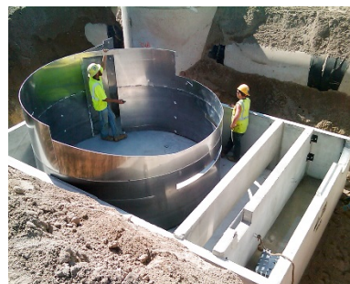
Figure 9-13 Installation of typical manufactured treatment device
