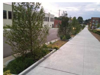
Figure 8-17 Vertical curbing adjacent to sidewalk
