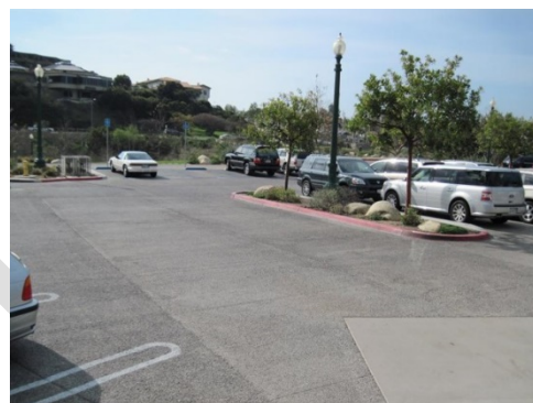
Figure 10-12 Permeable Parking Lot
