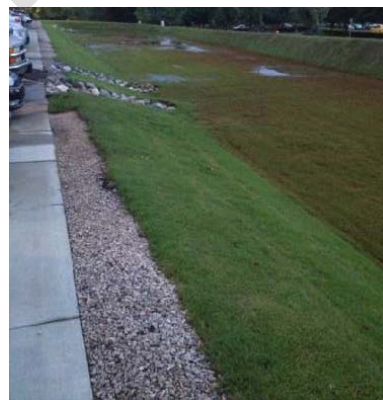
Figure 8-21 Gravel fringe flow spreader
