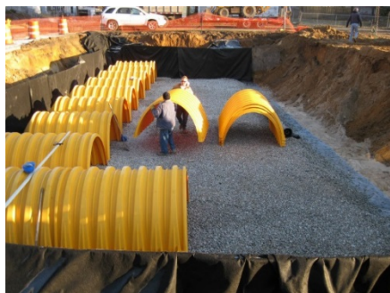
Figure 9-4 Infiltration Vault
