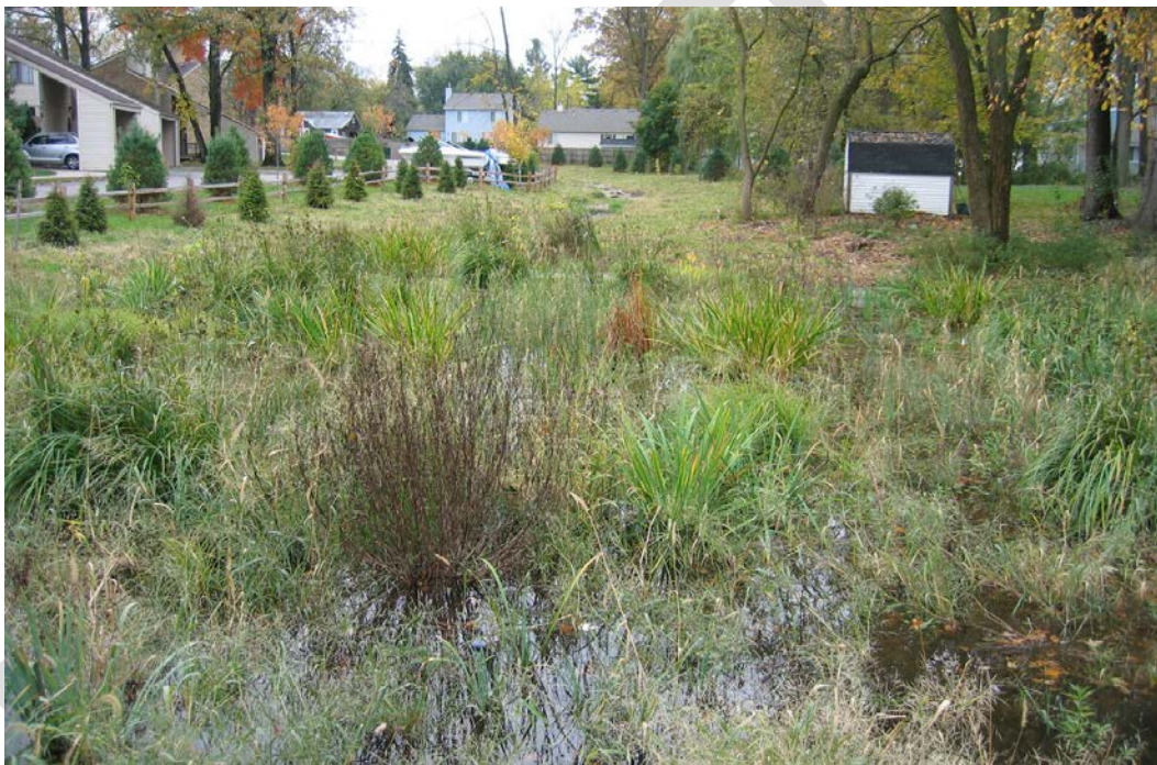
Figure 13-1 Example Surface Flow Stormwater Wetland
