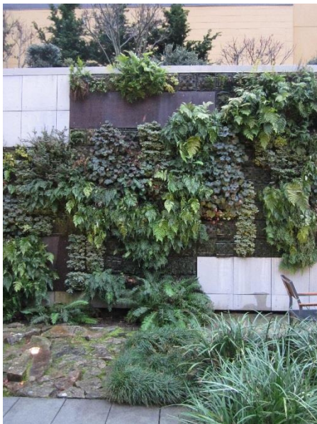
A “Living Wall” and bioretention area in Portland, OR.
