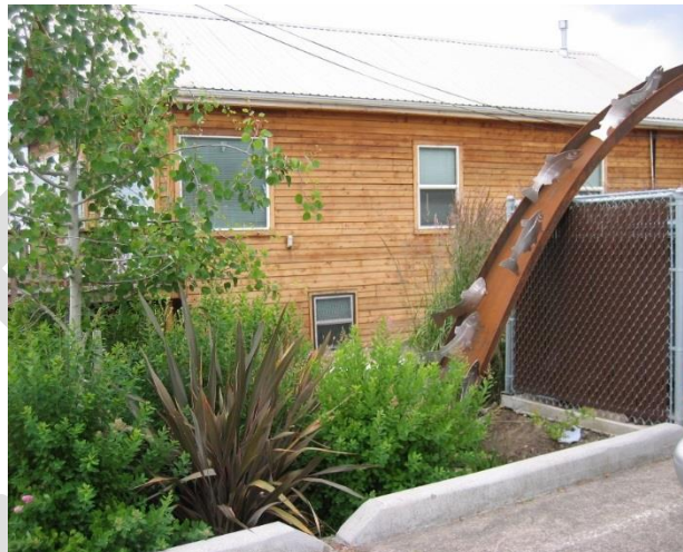
Artistic downspout into a bioretention area (Portland, OR)
