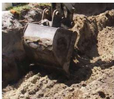
Figure 8-38 Scarifying soil with a toothed excavator bucket
