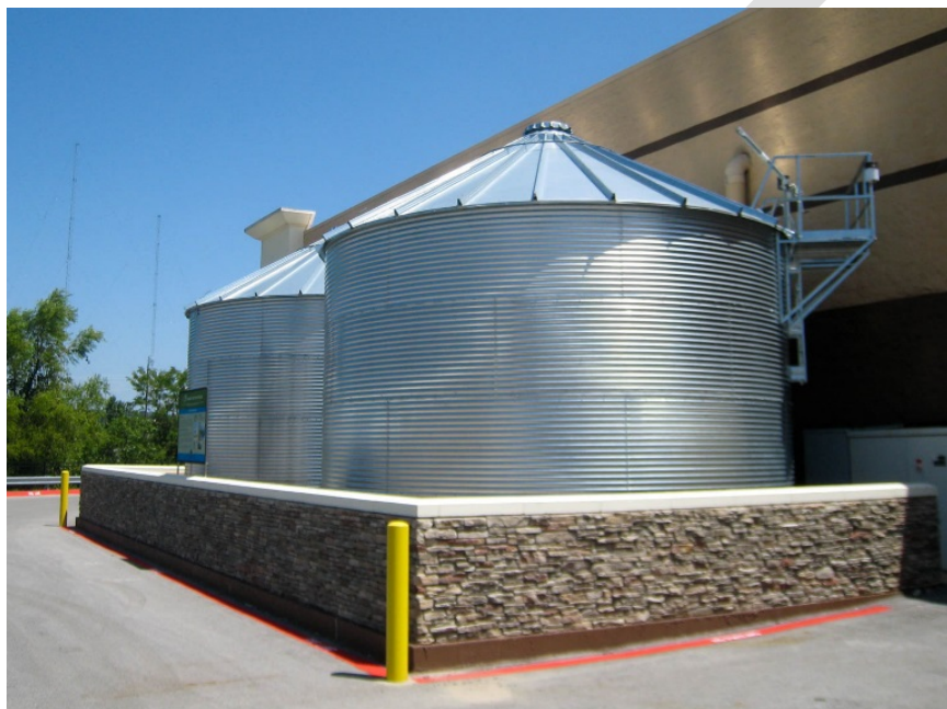
Figure 11-1 Cistern Example Used for Irrigation
