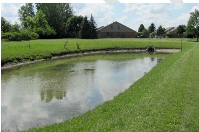
Figure 7-6 Detention with a Permanent Pool
