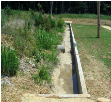
Figure 9-10 Typical level spreader
