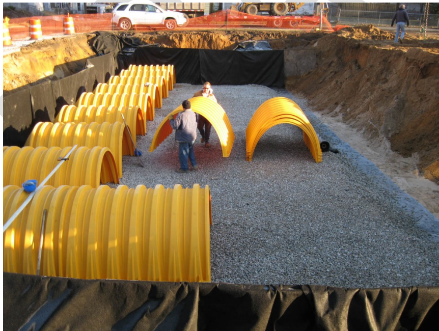
Figure 7-11 Subsurface Detention During Construction
