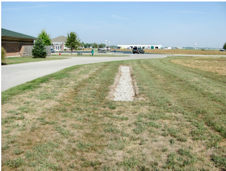
Figure 9-1 Infiltration trench installed adjacent to drive lane
