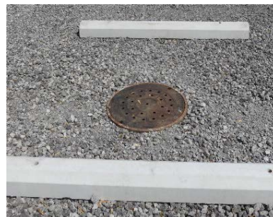
Figure 8-26 Permeable aggregate parking lot outlet structure
