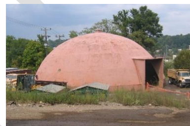
Covered material storage area
