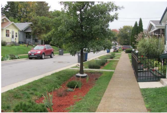
Figure 8-9 Linear Bioretention Along Roadway
