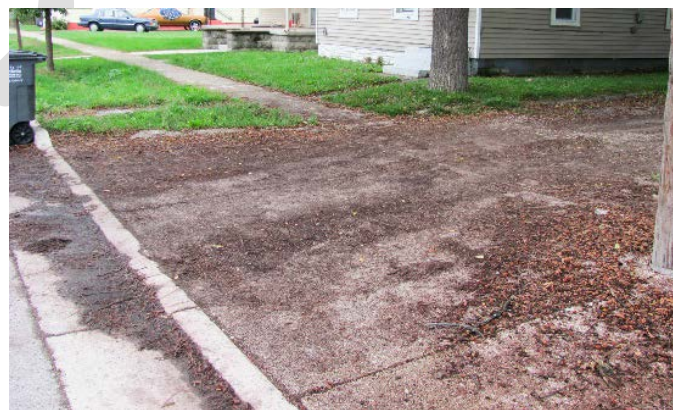
Figure 10-16 Permeable pavement with significant leaf litter
