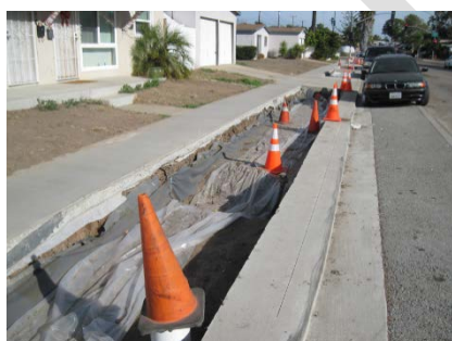
Figure 10-34 Protection of subgrade during construction
