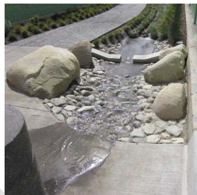
Figure 8-25 Armored inlet
