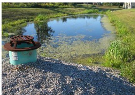
Retention basin with outlet riser
