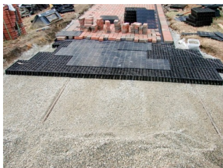
Figure 9-3 Infiltration Bed
