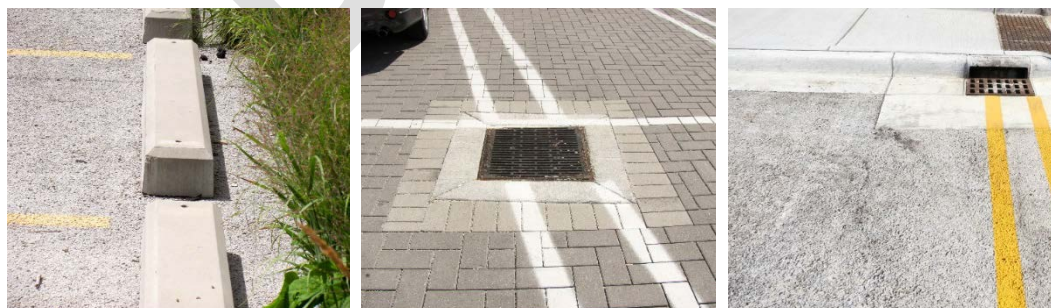
Pervious concrete parking; overflow conveyance to bioretention
