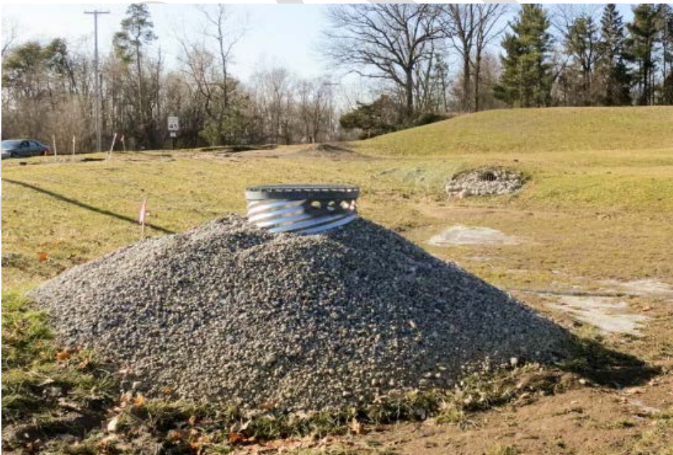
Figure 7-15 Typical Riser Pipe with Stone Jacket
