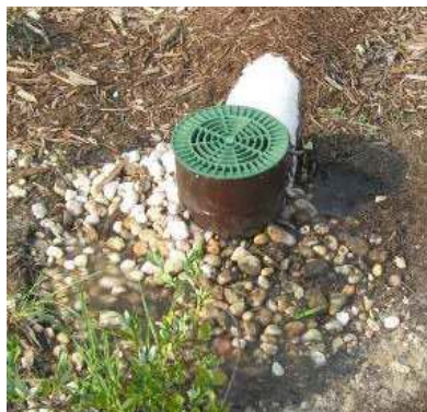
Figure 8-23 Upturned inlet
