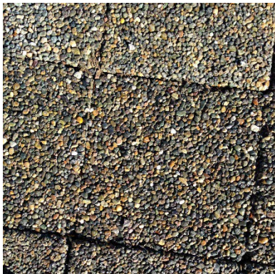
Figure 10-8 Example of Pervious Paver
