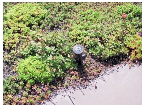
Figure 12-21 Overhead spray irrigation on vegetated roof
