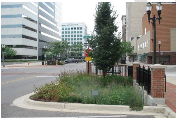
Figure 8-10 CBD Curb Extension Bioretention
