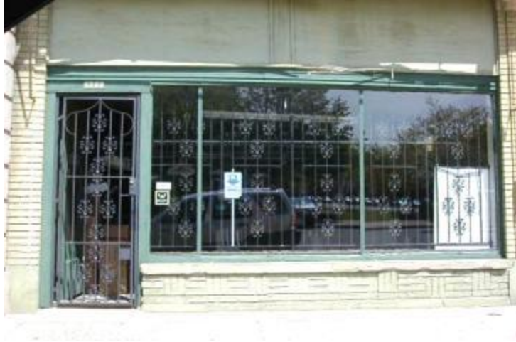
This storefront uses decorative security bars on the inside of the display windows.
