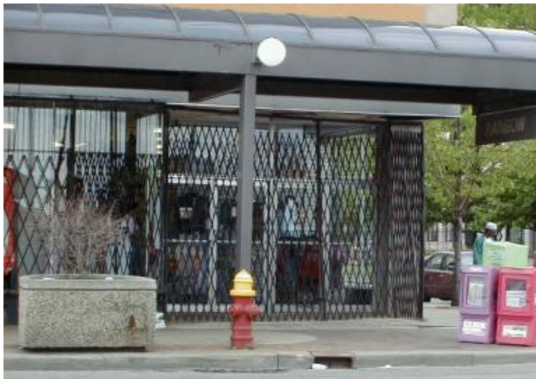
This storefront uses the scissor type security gate to protect the entrance and windows at night and is retracted during business hours.
