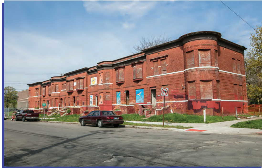
The Murray building in Southwest Detroit
