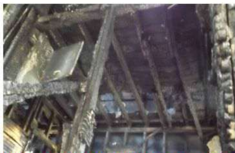
4509 CICOTTE REAR 2ND FLOOR JOISTS.JPG
