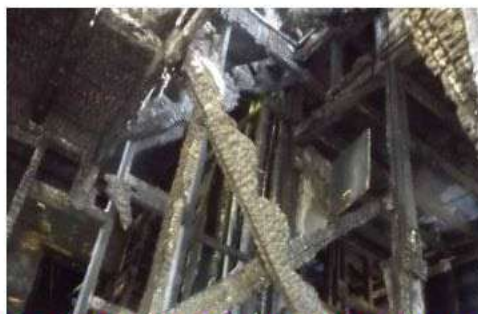
4509 CICOTTE REAR 2ND FLOOR STAIRS AND FLOOR.JPG
