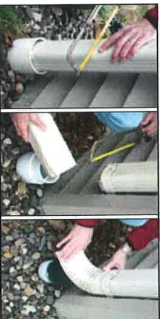
Downspout disconnect modification Source: http://www.granbuilding.ca
