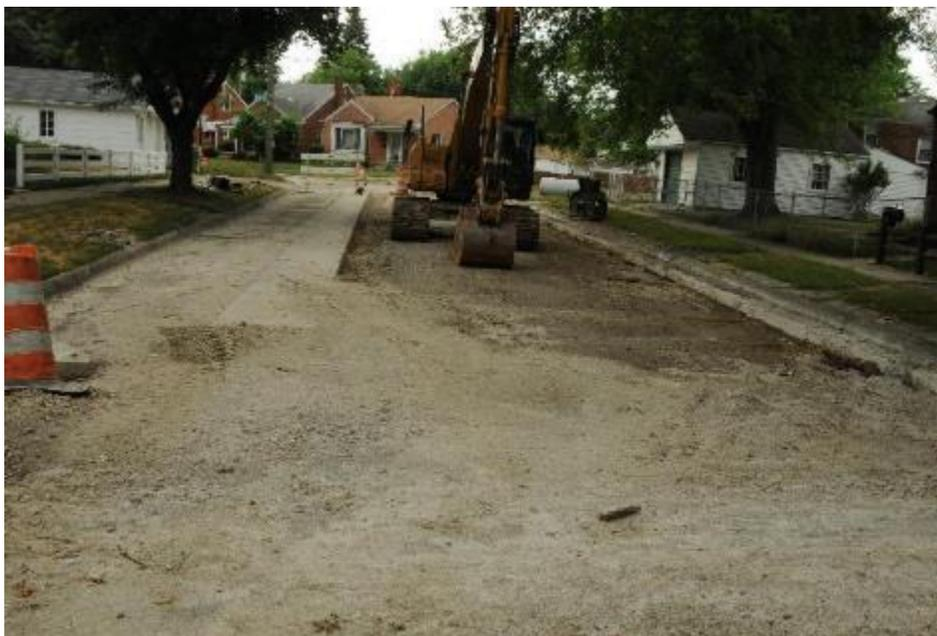
Tireman Phase I is also a component of PW6968. This phase consists of bioswales along the green space between the road and sidewalk that captures road runoff from Tireman Avenue. Overflow from the bioswales is conveyed to a separate storm sewer that runs east along Tireman where it is temporarily connected back into the combined sewer just west of Parkland Street. Phase I is currently under construction and is scheduled to be complete in fall 2016.
