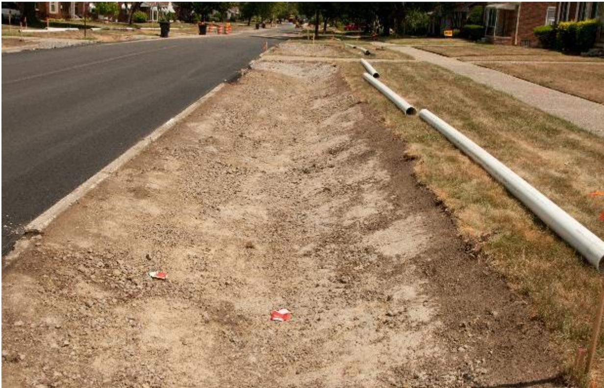
**Figure 27 Tireman Phase II Bioswale in Rouge Park Construction**
