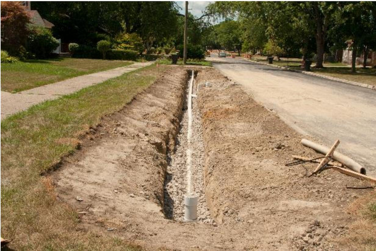
**Figure 26 Tireman Avenue Bioswale (Phase I) Final Grading Construction Photo**
