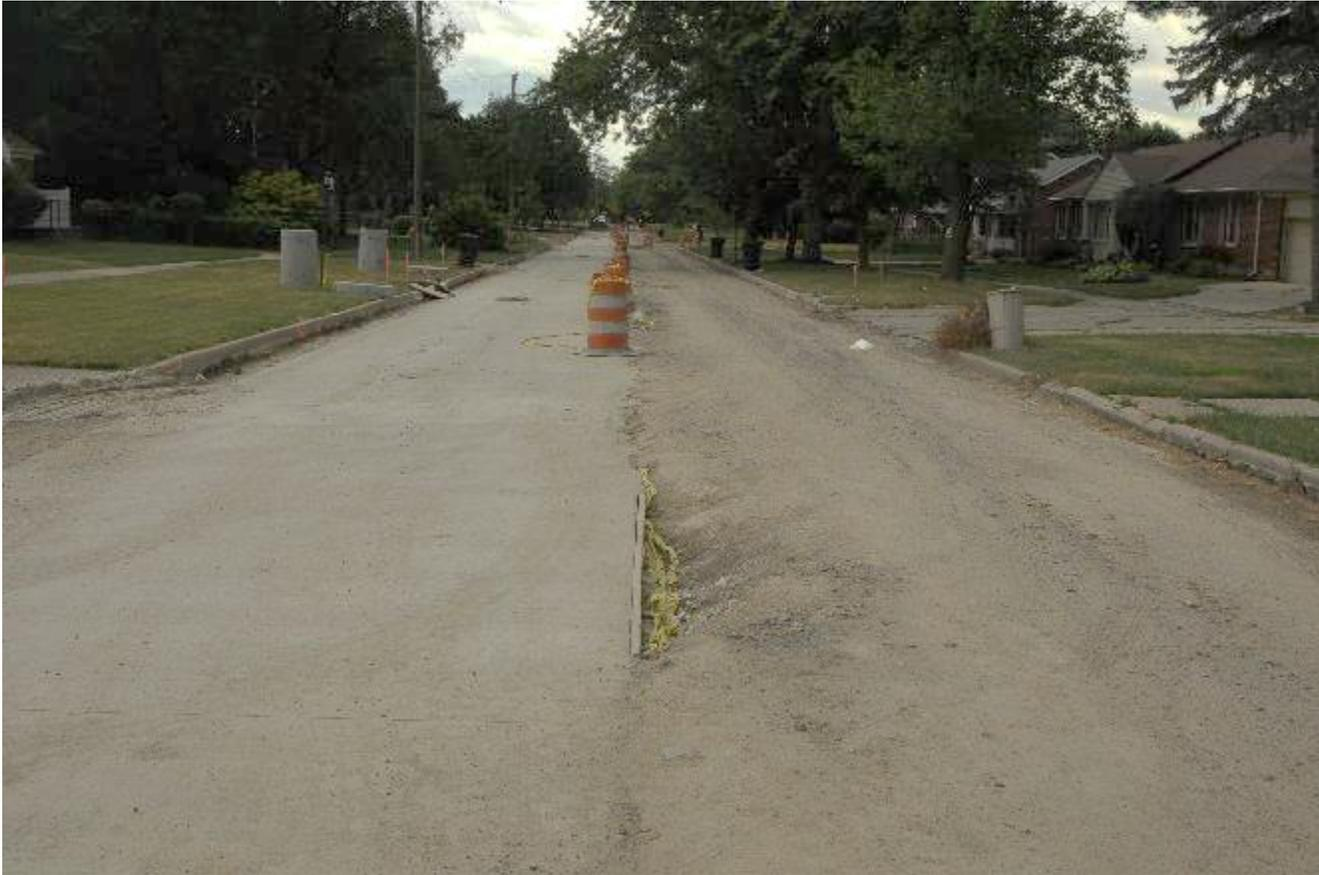
**Figure 25 Tireman Avenue Bioswale (Phase I) Underdrain Construction Photo**
