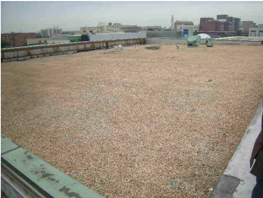
Detroit Institute of Arts Roof Area
