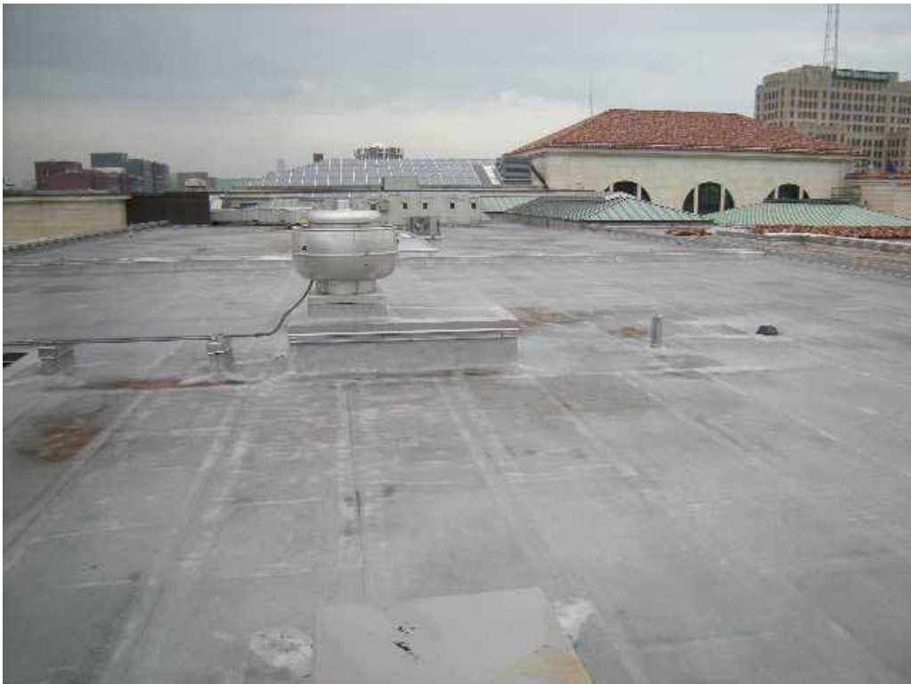
Detroit Institute of Arts Roof Area
