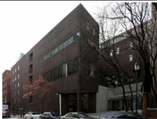
Former Balch Institute
