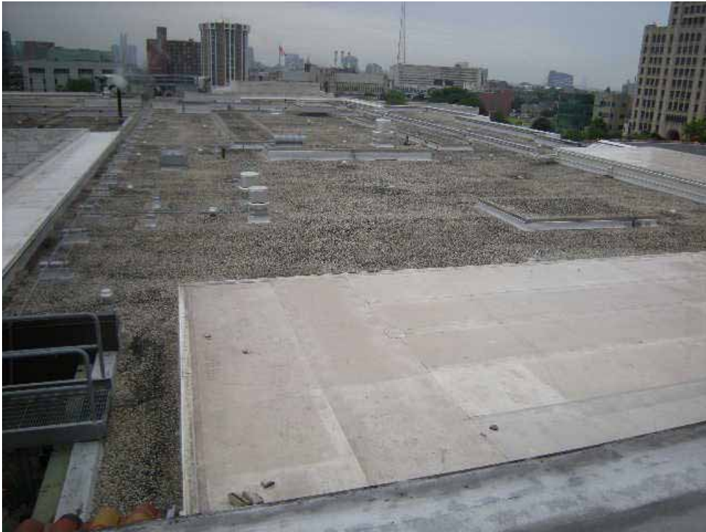
Detroit Institute of Arts Roof Area
