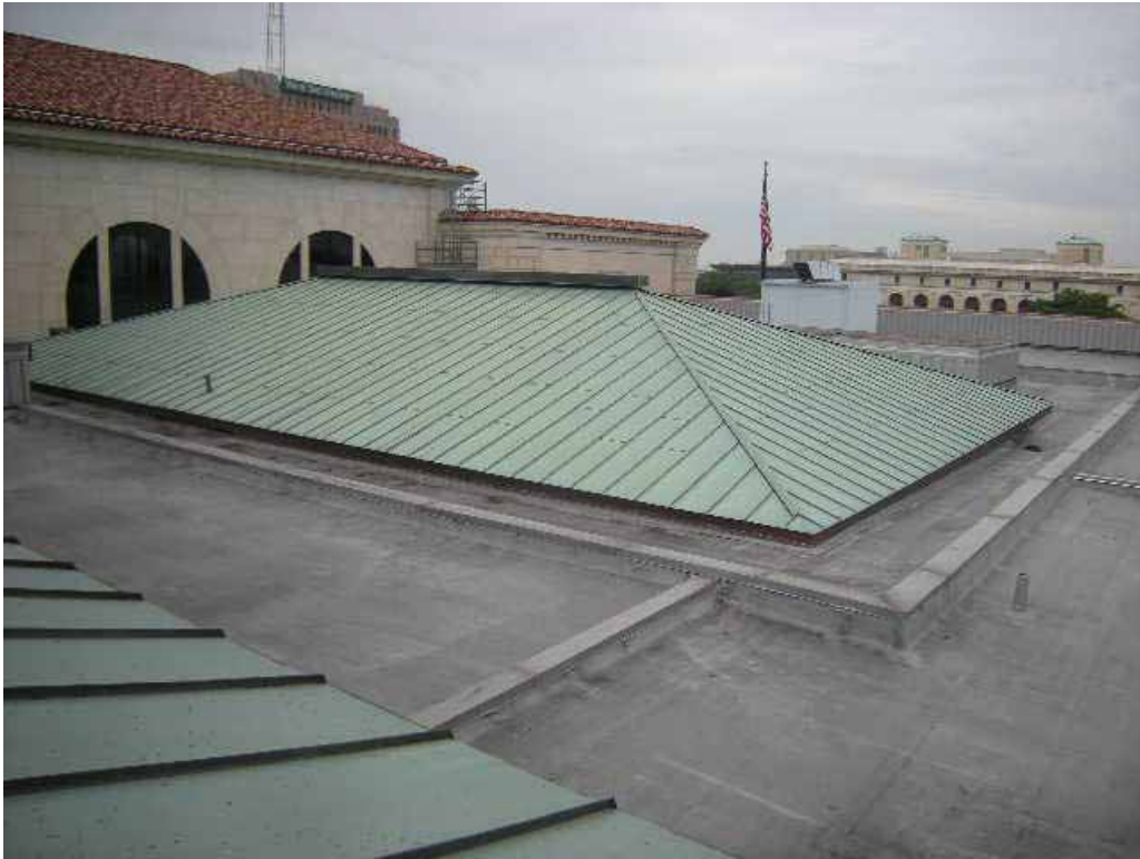
Detroit Institute of Arts Roof Area
