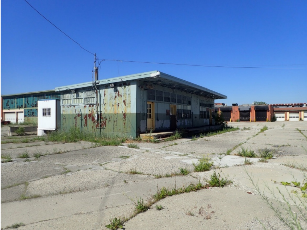
Figure 41. 14044 Schaefer Highway, Coolidge Fare Box House
