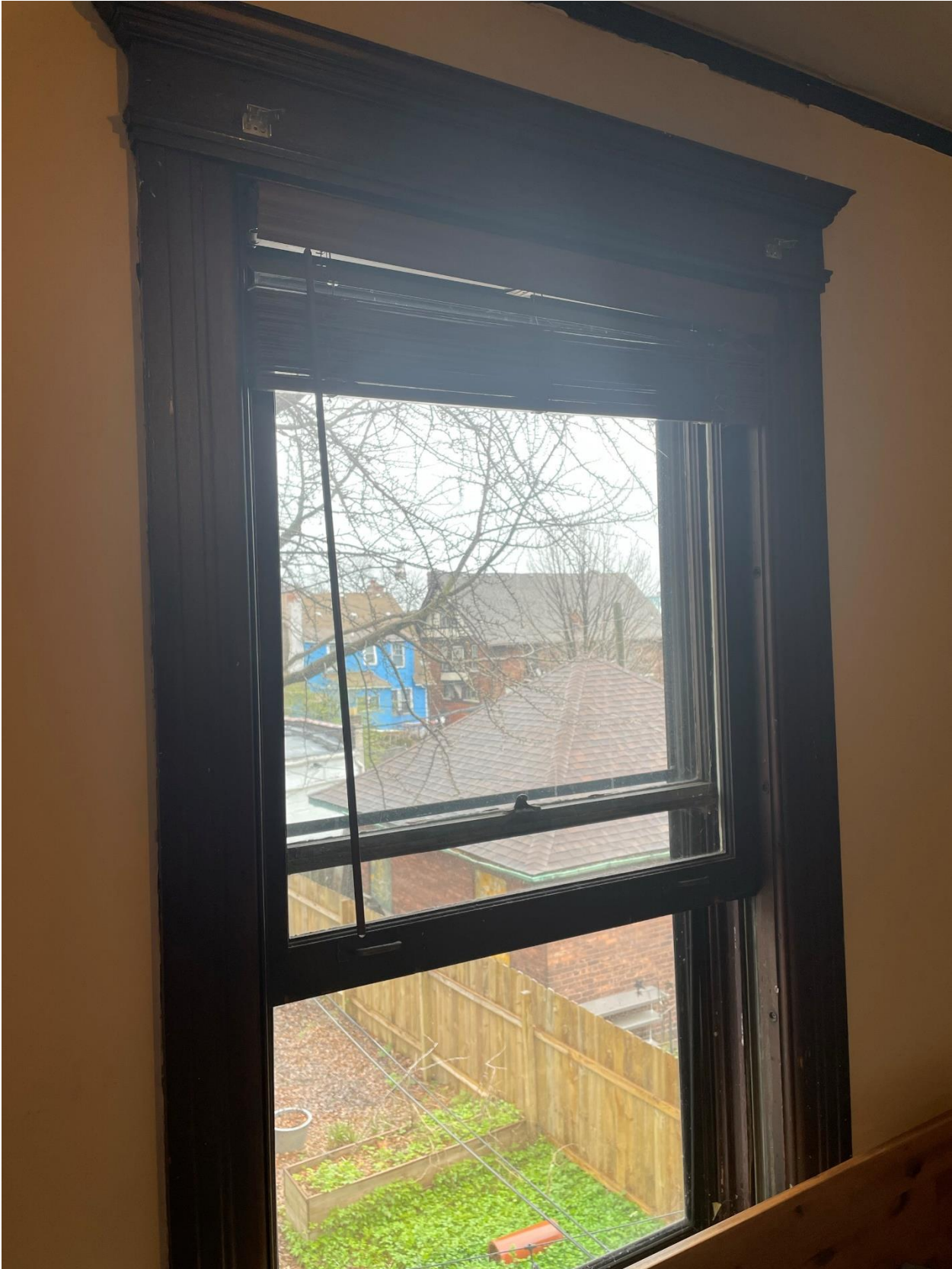
First floor West Window #14
