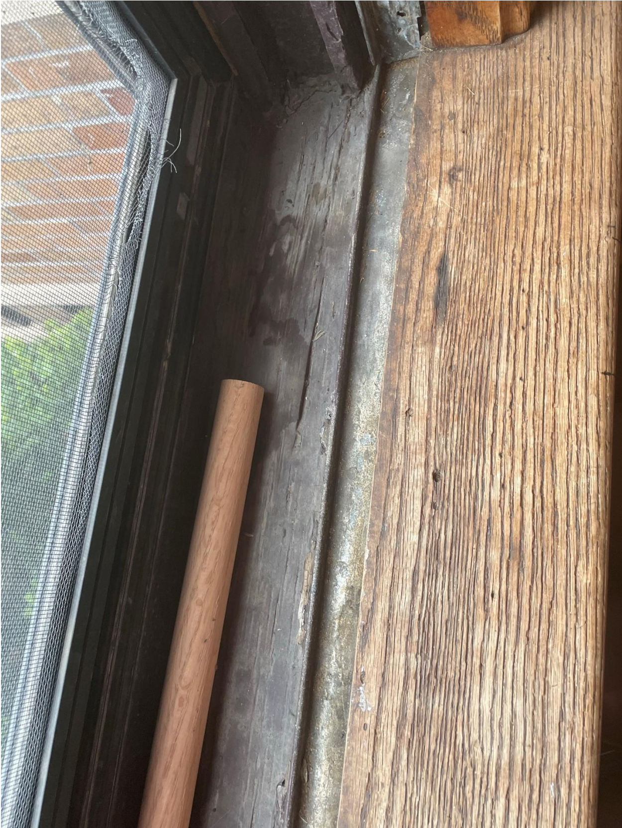
Window #1 - Waterdamage
