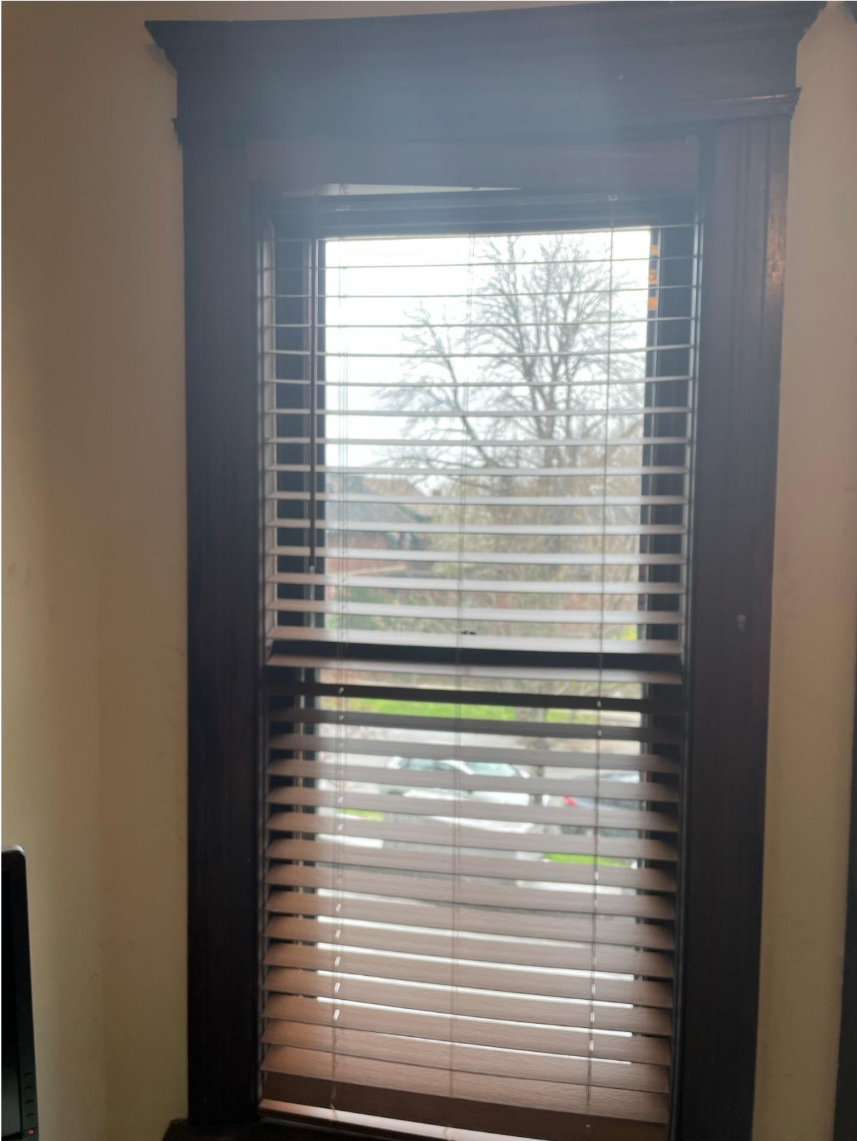
First floor West Window #10
