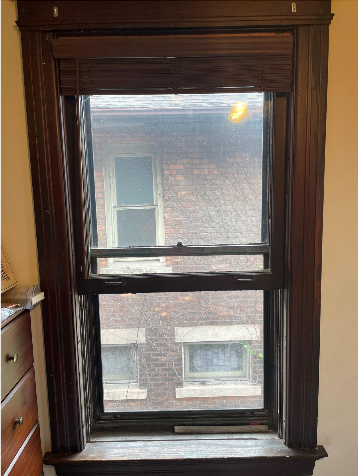
First floor West Window #13
