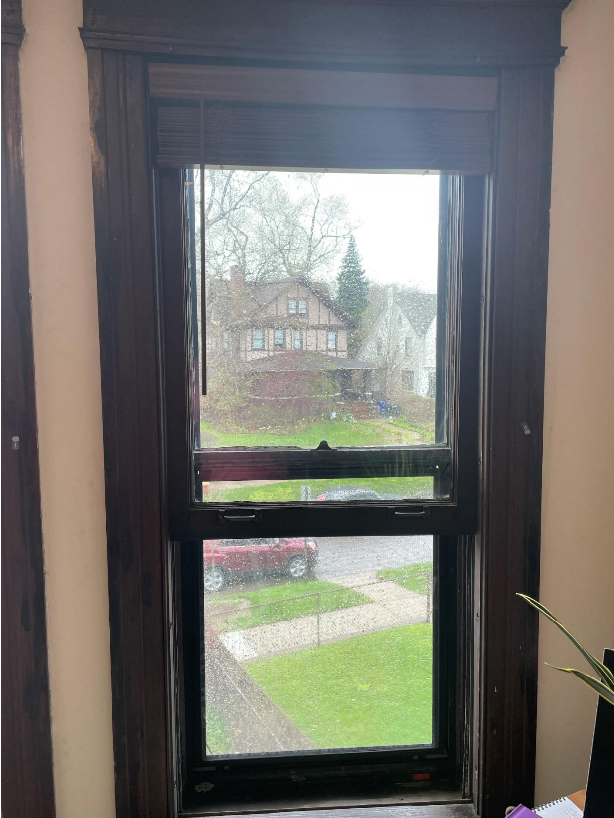
First floor West Window #12
