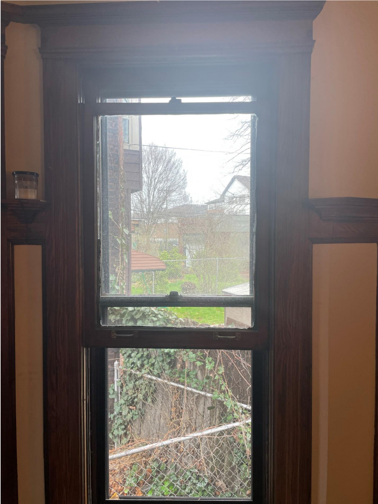
First floor West Window #7
