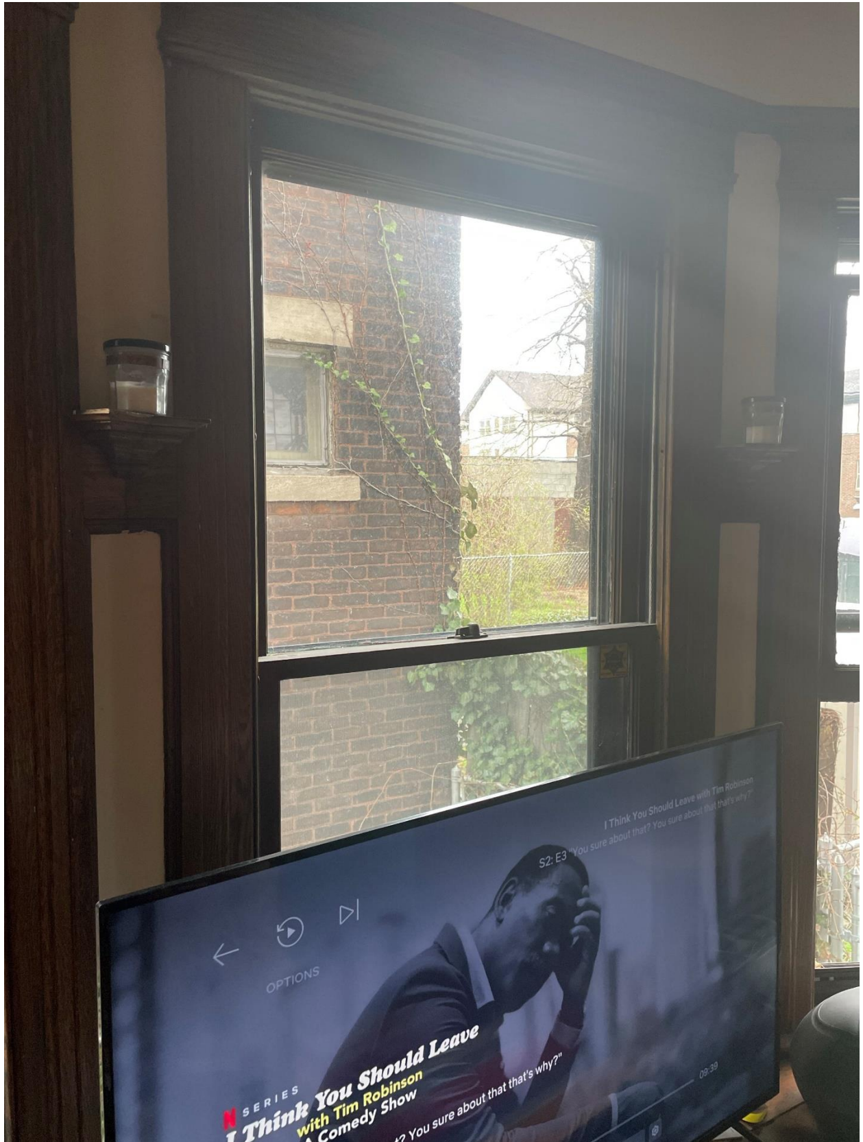
First floor West Window #6
