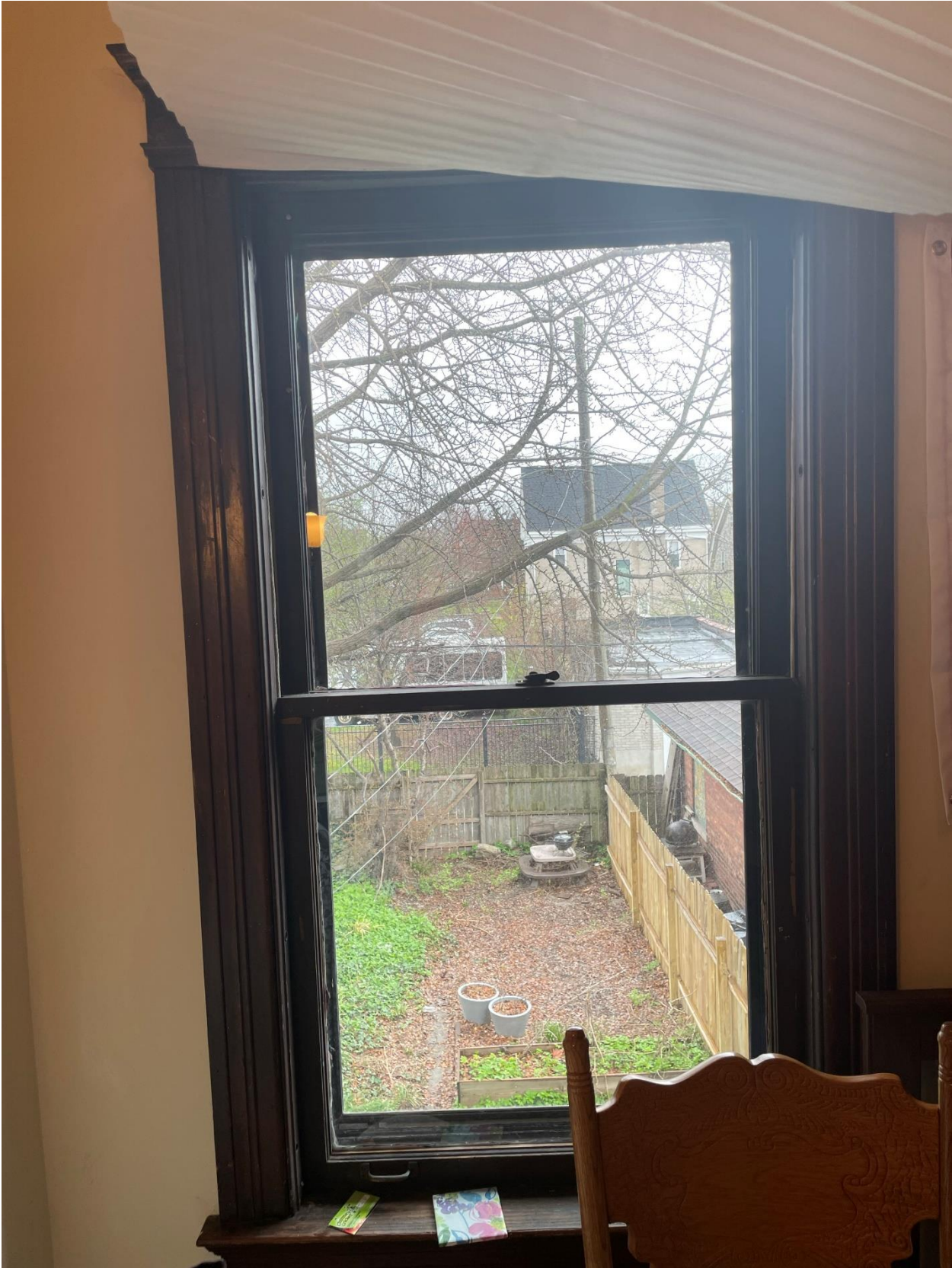
First floor West Window #15
