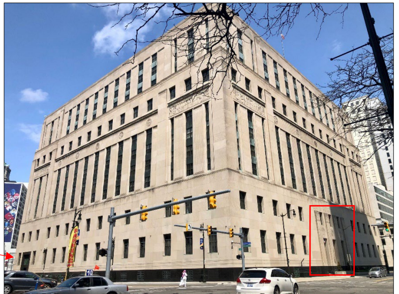
View of southwest corner of building – (l) Washington Boulevard and (r) Fort Street. The building's secondary entrance is centrally located on Fort Street. Staff photo, April 18, 2024.
