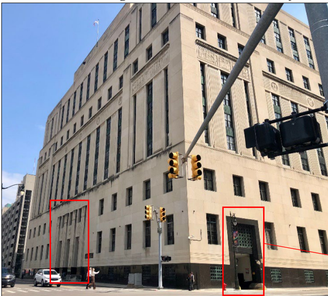
View of northwest corner of building; (l) W. Lafayette Street and (r) Washington Boulevard. The building's primary entrance is on W. Lafayette and one underground garage entrance is at Washington Boulevard. Staff photo, April 18, 2024.
