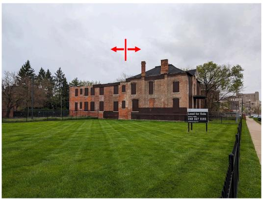
Distant view of left side (east) elevation, looking towards the west. The two construction phases (original mansion and 1920s addition) are easily read here, divided by the vertical red line. Staff photo, April 23, 2024.
