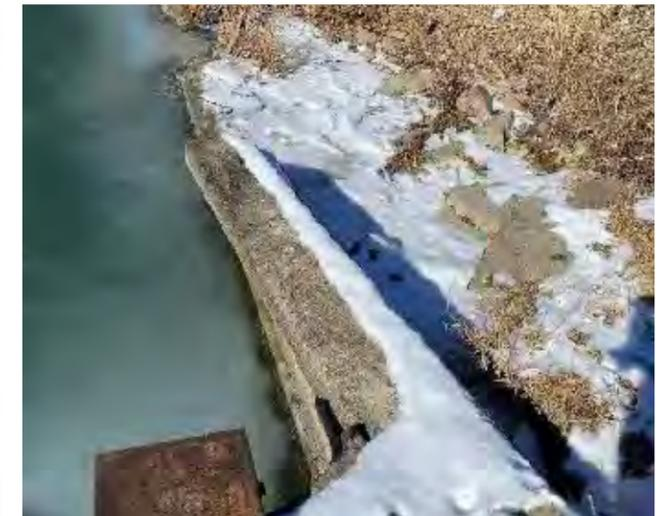
Noted deterioration of concrete seawall
