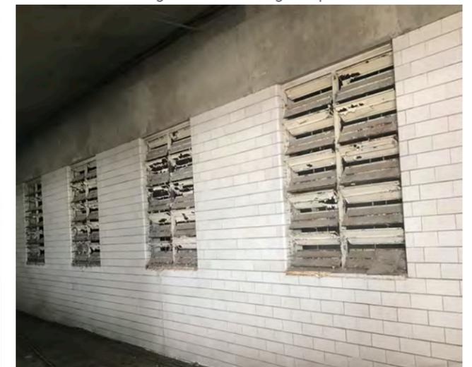
Damaged air vents in the lower level
