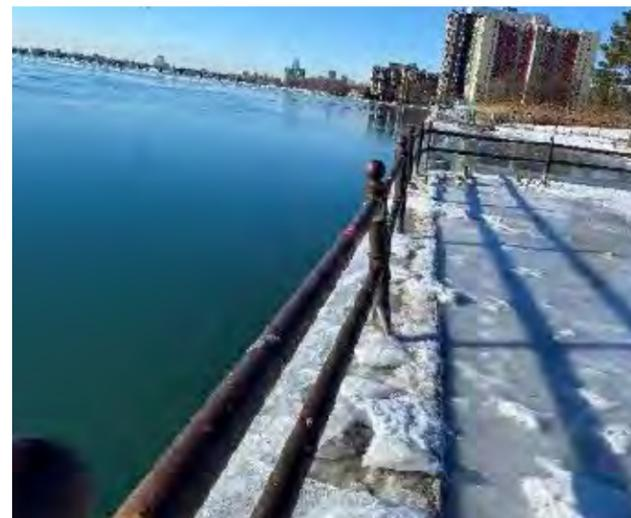
Existing concrete and steel sheet pile wall, leaning railing sections and flooding noted
