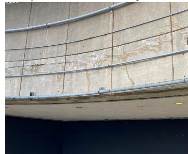
Severe horizontal cracking and significant moisture in the lower level.
