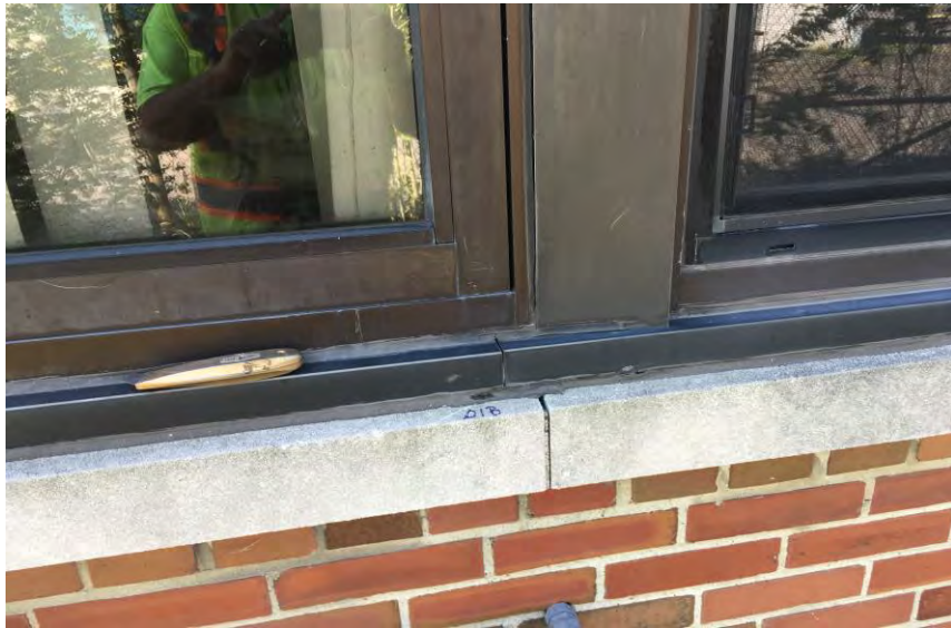
Sample #1 a Brown Caulk of Terminal Building
