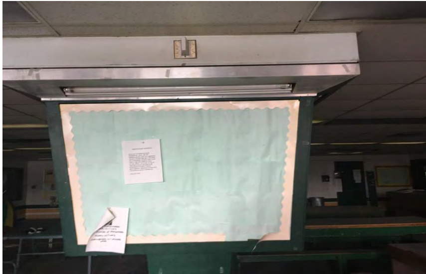
Message Boards in the Terminal Building
