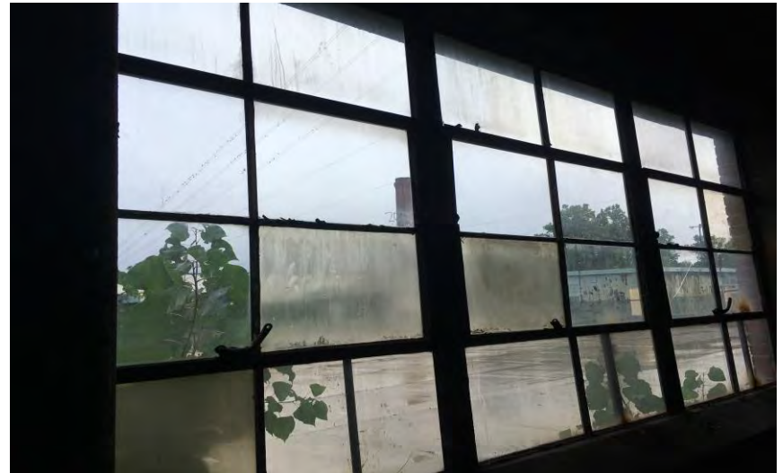
Window Glazing in the Boiler Building Samples #2 & #3
