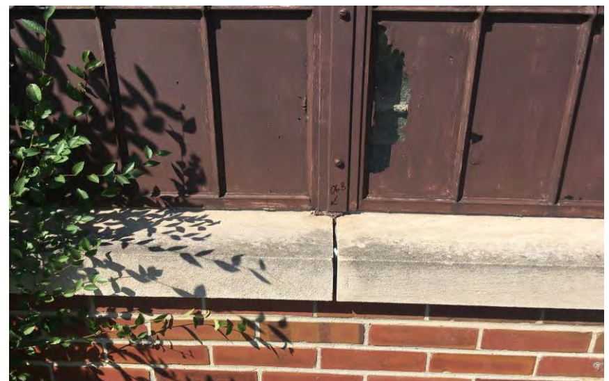
Sample #6 Painted Caulk East side of Terminal Building
