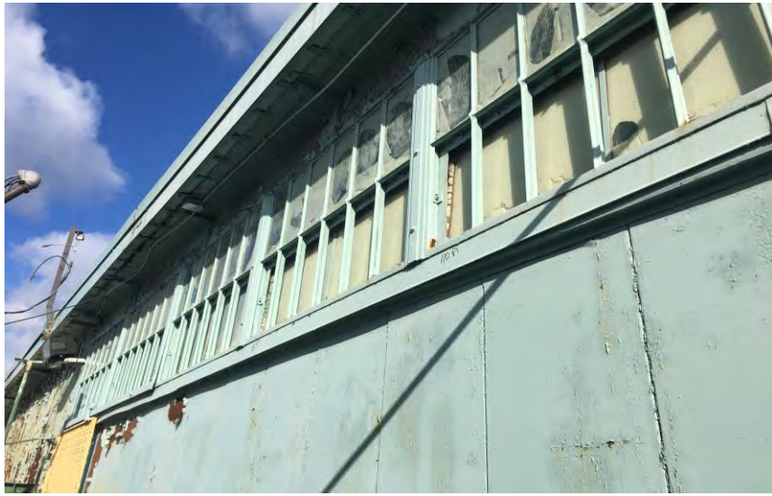
Window Glazing on the Fare Box Building Sample # 40
