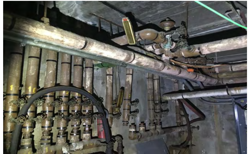
Aircell Insulation and Mercury Thermometers in the Basement to the Tunnel in the Terminal Building
