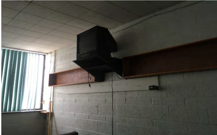
TV on the 2 nd floor of the Terminal building
