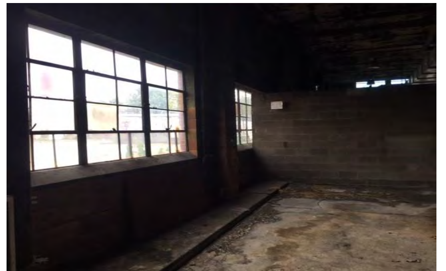
Window Glazing in the Bus Garage Sample #20 Room BB1118
