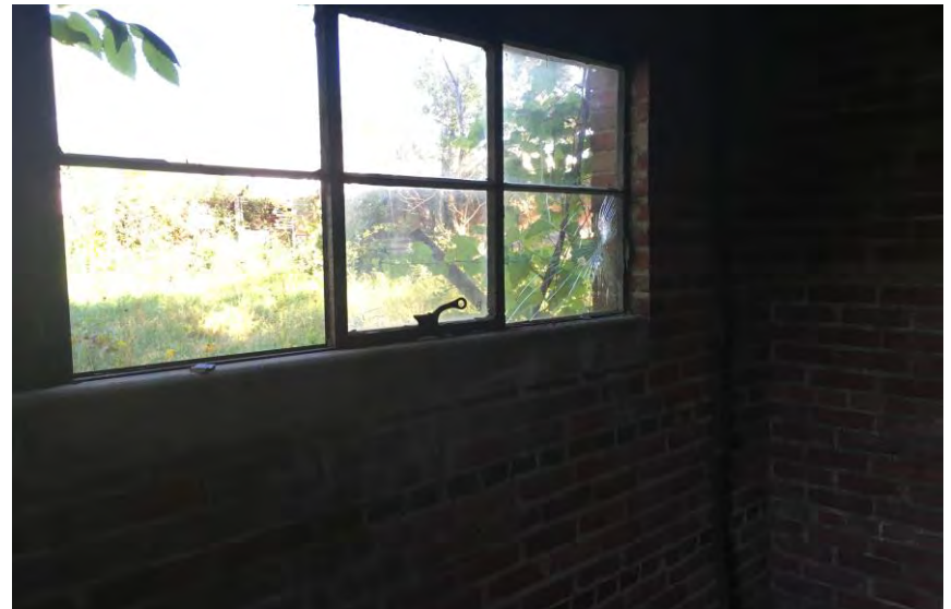
Window Glazing in the 1 Story Brick Building Sample # 38
