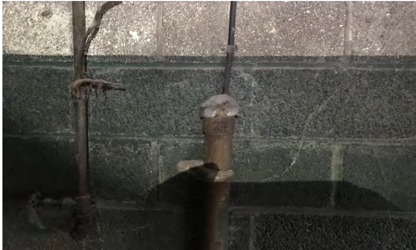
Sealant on top of Conduit Sample #27 Carriage Storage Bay #4
