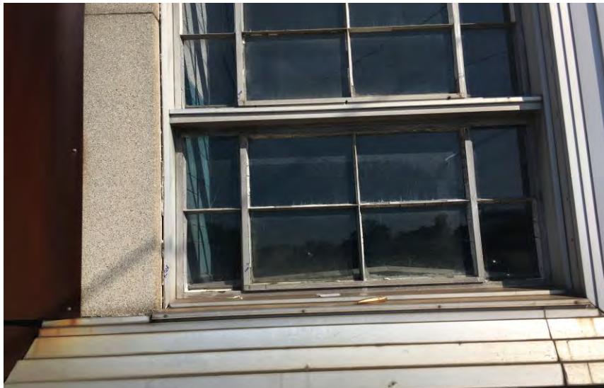
Sample # 2, 3 and 4 Caulk, Gray and White Window Glazing on Terminal Building
