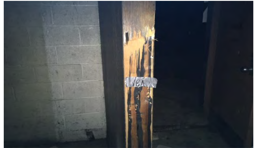
Paneling Mastic in the Bus Garage Building Sample # 18 Room BB1114
