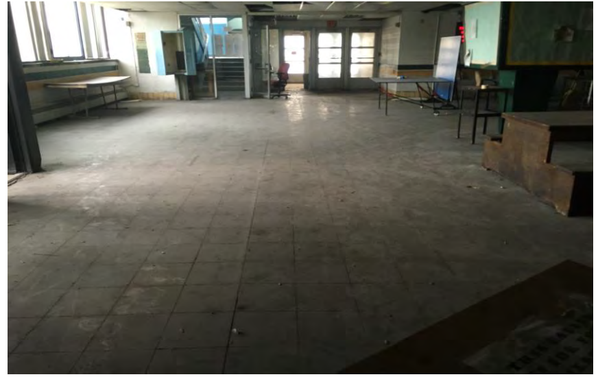
Sample #23 9"x 9" VFT under the 12" Tiles in Terminal Building
