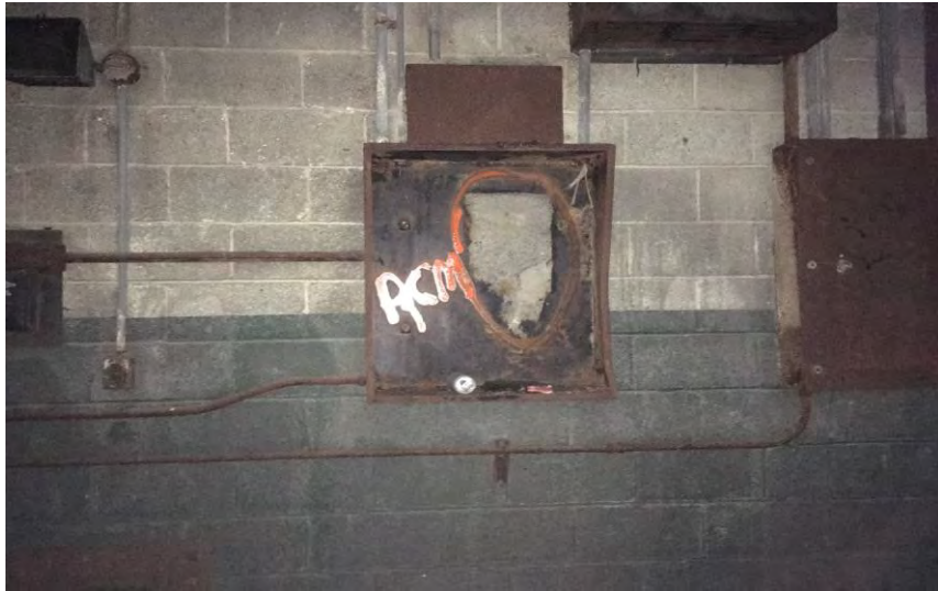
Asbestos Paper in Electrical Boxes in the Bus Garage, 1 of 9, Sample #7 and Sample #21
