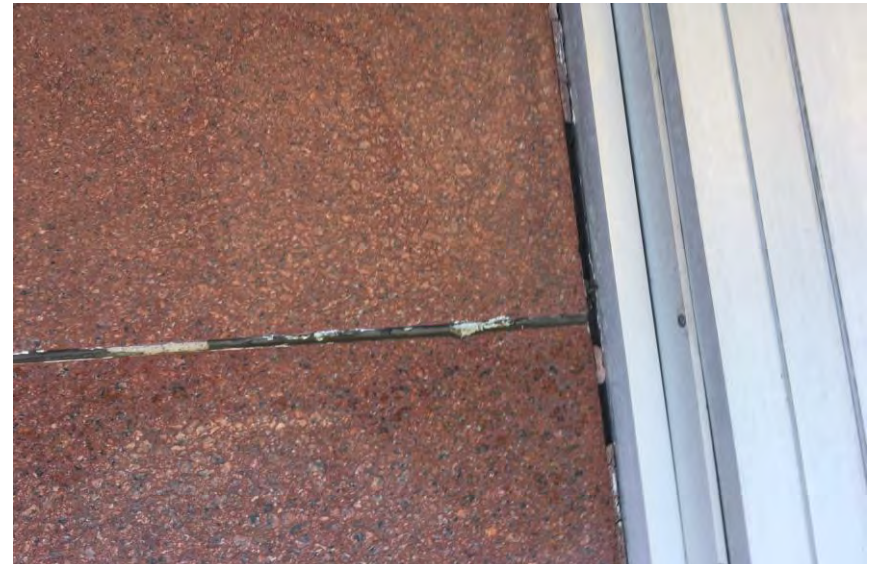
Sample #5 Red Caulk on the South side of Terminal Building
