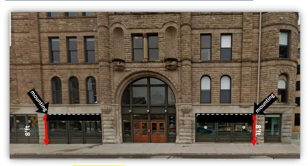
Fabric Awning <mark>(Grand River)</mark> Awnings to be Mounted to Inside Window Frame 8ft height is allowed from Grade to Top of Awning Area Note: (2) Fabric Canopy Located at Over Windows Southeast Facade
