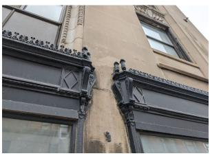
Site Photo 4, by Staff March 27, 2024: (west elevation) showing cast iron header detail over storefront, and newer storefront window units fitted carefully into the original frames.
