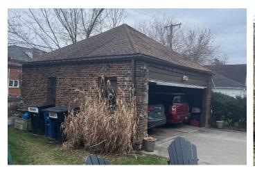
*Site Photo 3, by Staff March 27, 2024: (North) side elevation of garage, showing some step cracks in the masonry.*
