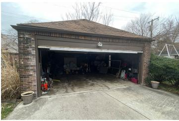
Site Photo 2, by Staff March 27, 2024: (West) front elevation of garage, showing foundation cracks, bowing of center roof, and some efflorescence and cracks in the masonry.
