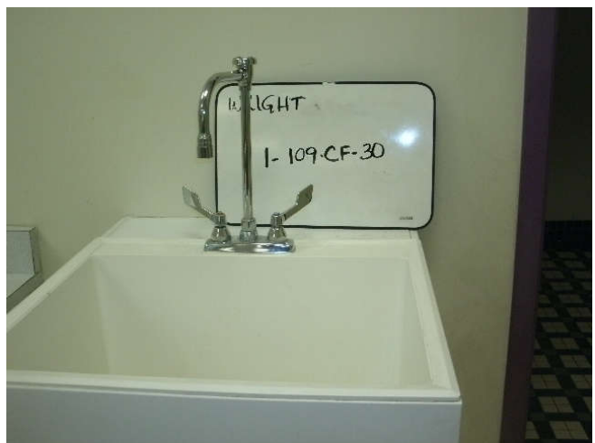
Photo 30: Classroom faucet, located on the 1st floor, in room 109.
