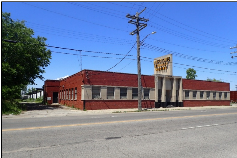
Figure 20: O.H. Frisbie Moving and Storage Building
