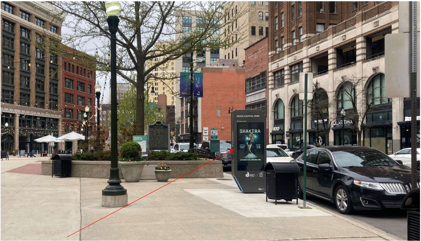
Electronic kiosk #1, installed within without HDC approval, facing north. Staff photo taken on 4/22/2024
