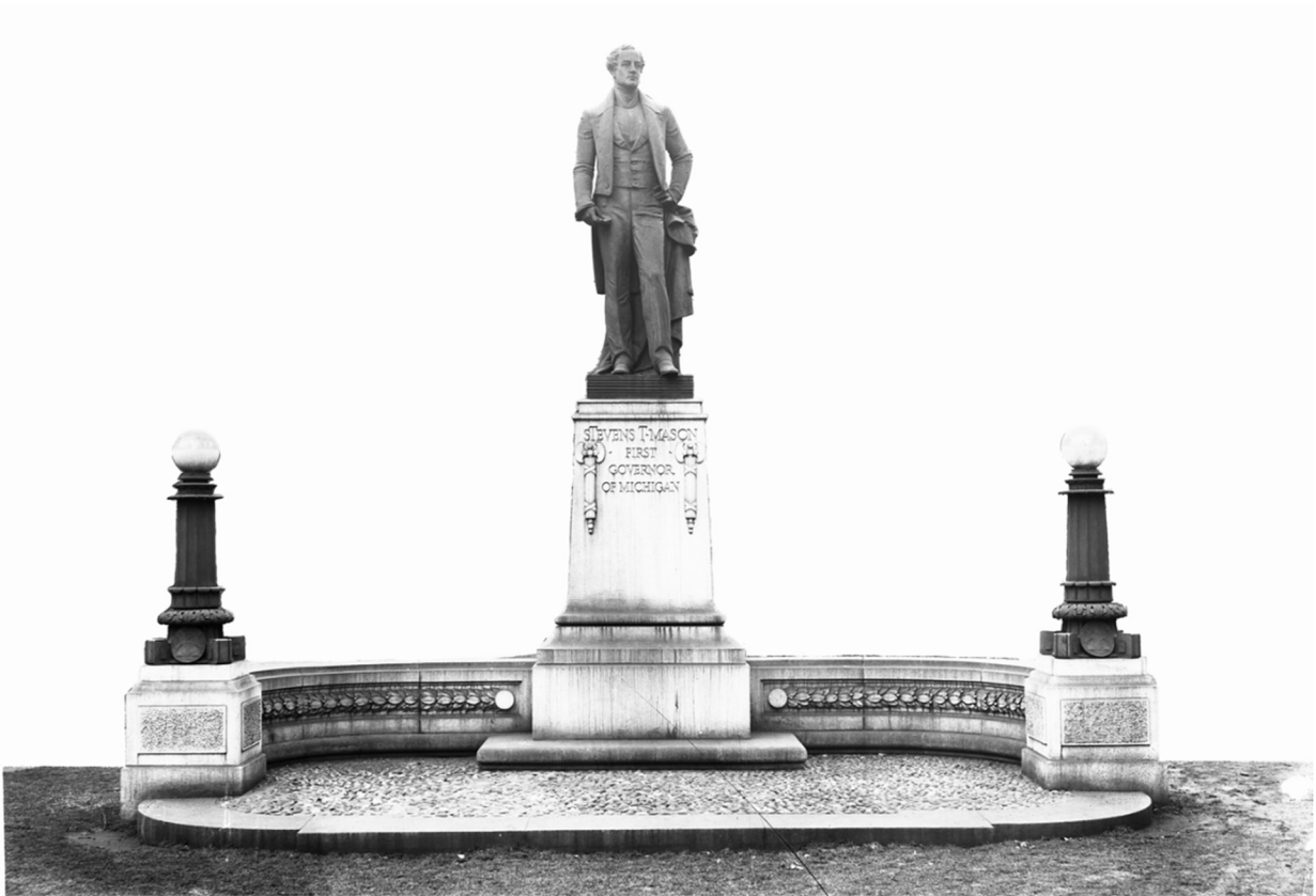
Photo of the Mason monument, showing original masonry floor, balustrade/exedra, and light fixtures. These framing elements were removed ca. 1955 when the monument was moved from its original location at the north end of the park to the south end of the park to accomodation the location of a new bus station within the park
