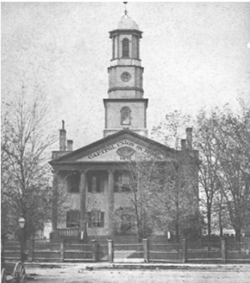
The former Capitol Building after it was repurposed for use as the Capitol Union School, ca. 1870
