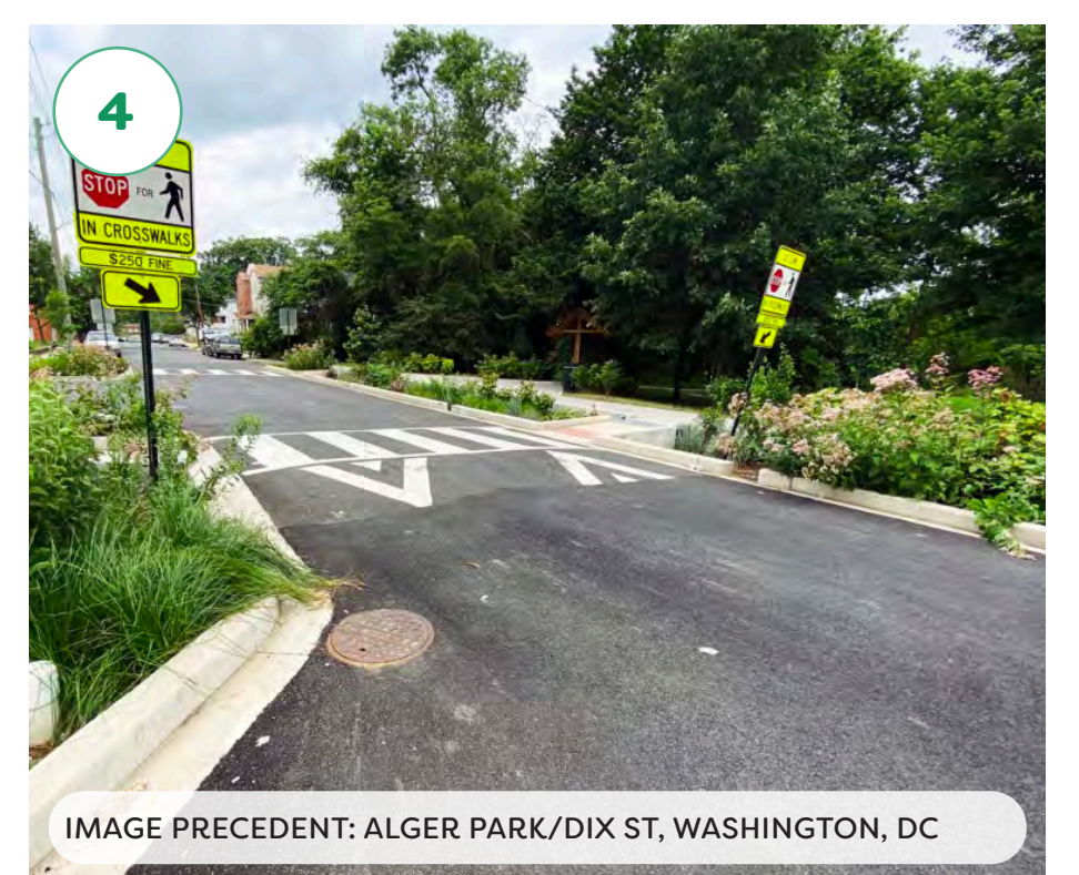
NEW STORMWATER CONNECTION
