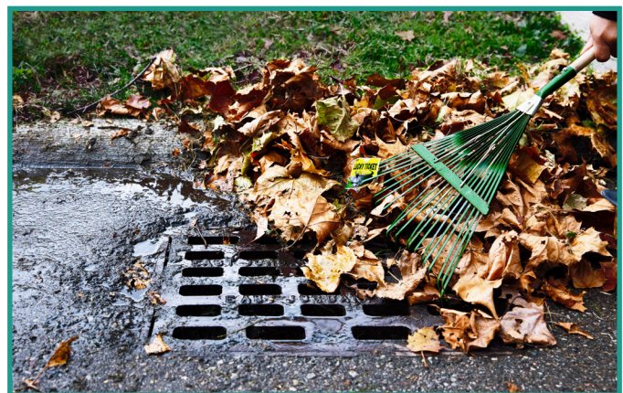
Clean above and around catch basins - reduce the potential for neighborhood flooding
