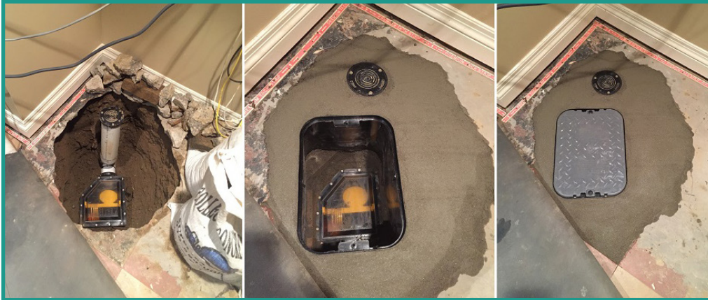
Steps involving a backwater valve installation
