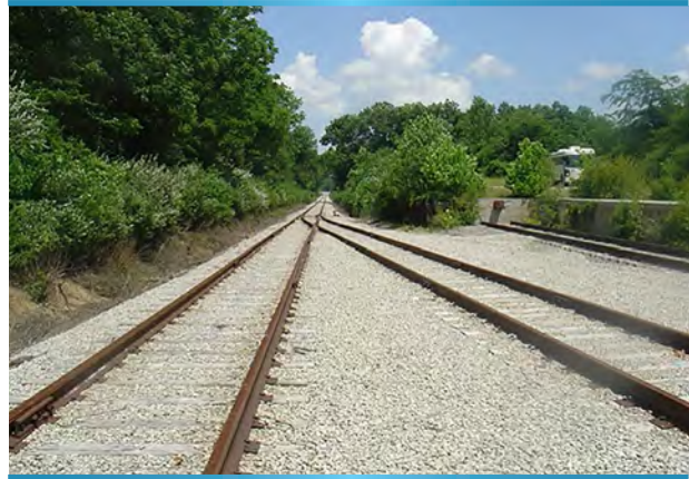
Pervious Railroad Ballast
