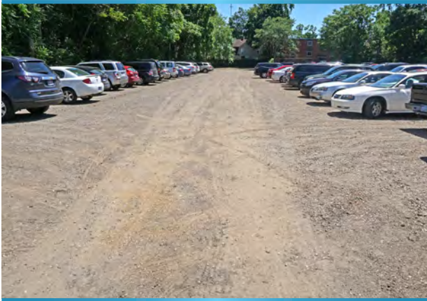
Compacted Gravel Parking Lot
