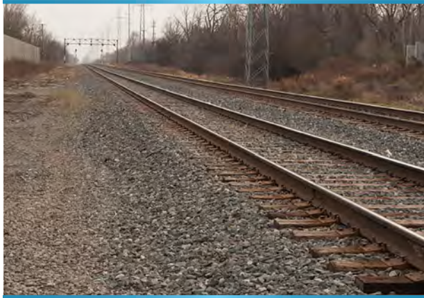
Pervious Railroad Ballast
