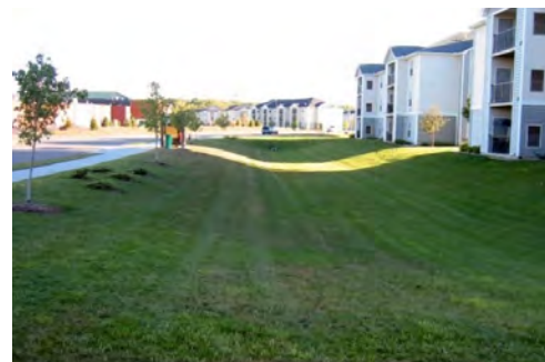
Dry Detention Basin
