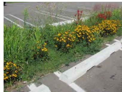
Bioretention between Parking Lot Aisles
