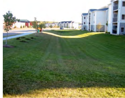
Traditional Dry Detention Basin
