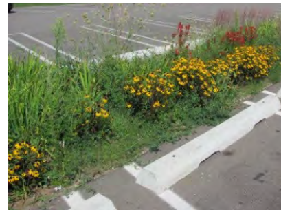
Bioretention between Parking Lot Aisles
