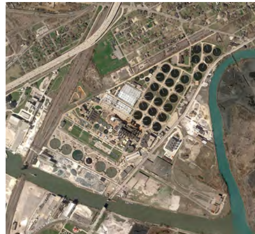
Detroit’s Wastewater Treatment Plant
