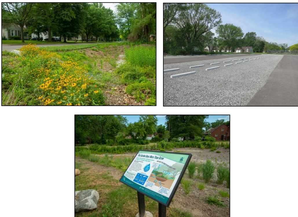
Figure 8 Stoepel Park Bioretention and Parking Area
