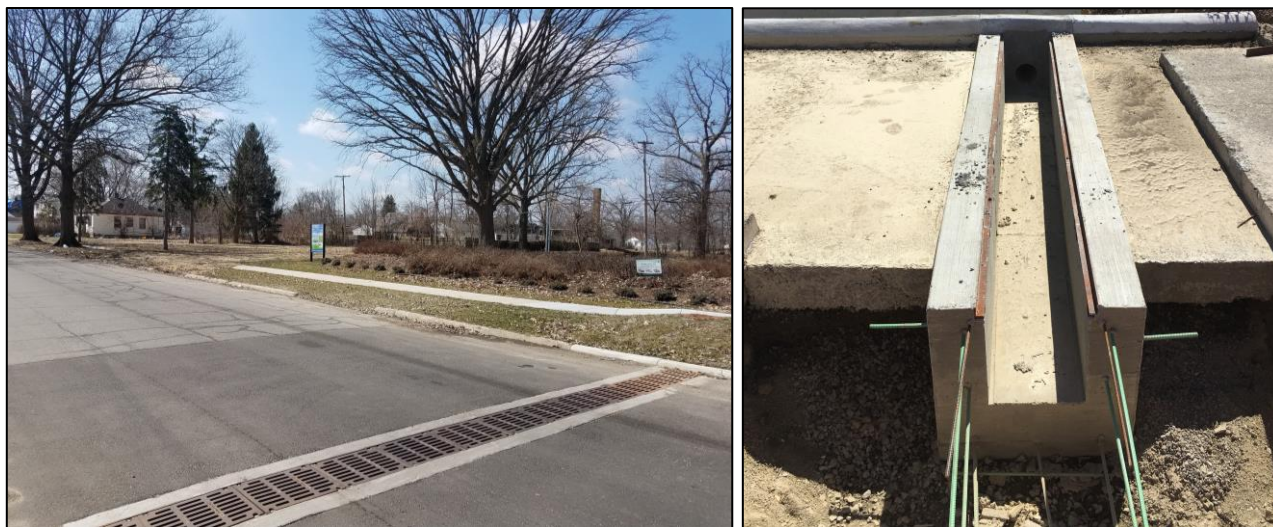
Figure 16 Eco Site Retrofits
