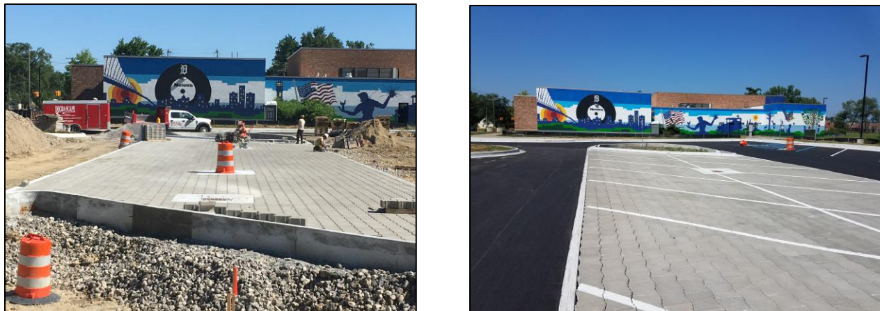
Figure 12 Crowell Recreation Center Parking Lots
