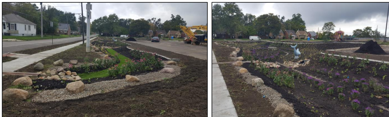
Figure 15 O'Shea Park Construction
