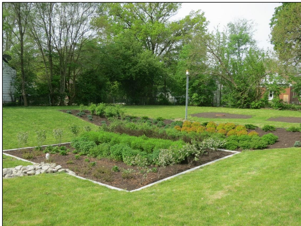
Figure 7 Evergreen Vacant Lot Bioretention – Site
