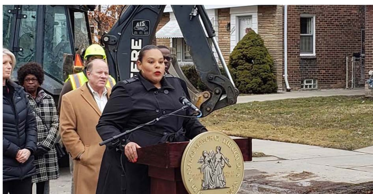
DWSD Deputy Director & Chief Engineer Palencia Mobley, P.E., stands with Mayor Mike Duggan, Councilman Andre Spivey and members of the community at a groundbreaking on March 5, 2020 to launch the City's first neighborhood-wide projects to upgrade the water and sewer systems. The groundbreaking was held in the Cornerstone Village neighborhood on the city's eastside.
