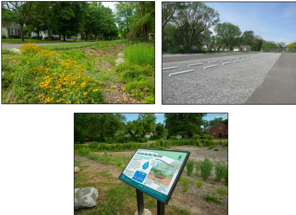
Figure 7 Stoepel Park Bioretention and Parking Area
