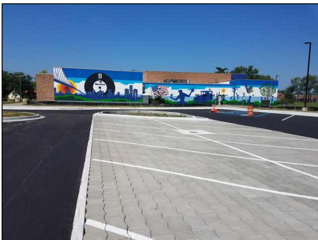
Figure 1 Construction Completed in FY2019 Crowell PaveDrain (left) and O'Shea (right)
