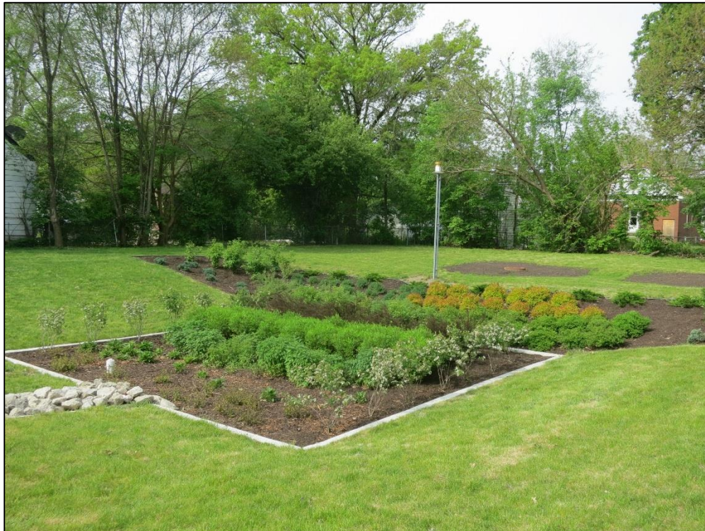
Figure 6 Evergreen Vacant Lot Bioretention – Site
