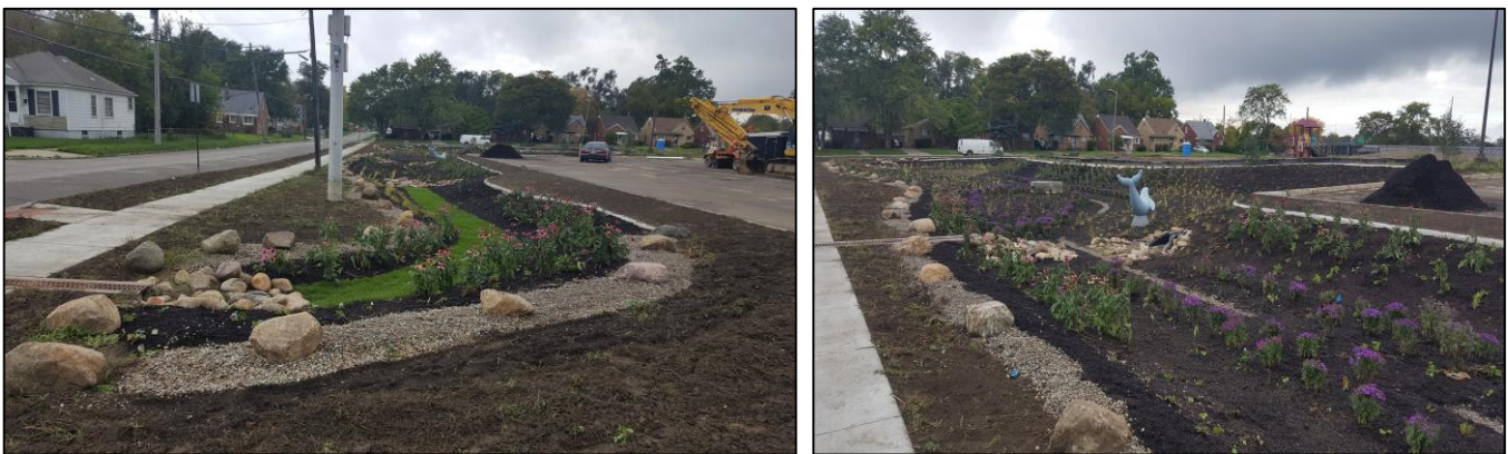
Figure 14 O'Shea Park Construction
