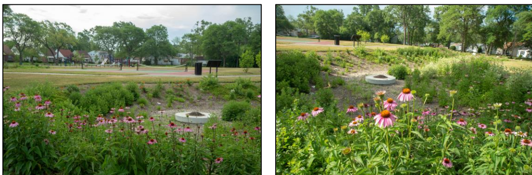
Figure 8 Liuzzo Park Bioretention Improvements
