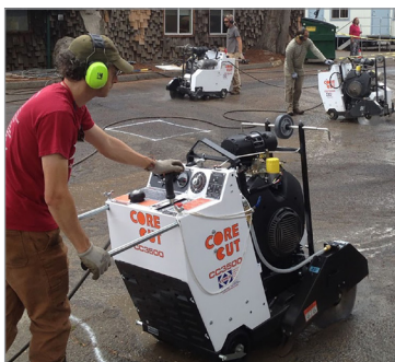
Concrete cutter to remove pavement Photo credit: Eric Rosewall - Depave.org
