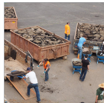
Recycling pavement Photo credit: Eric Rosewall - Depave.org
