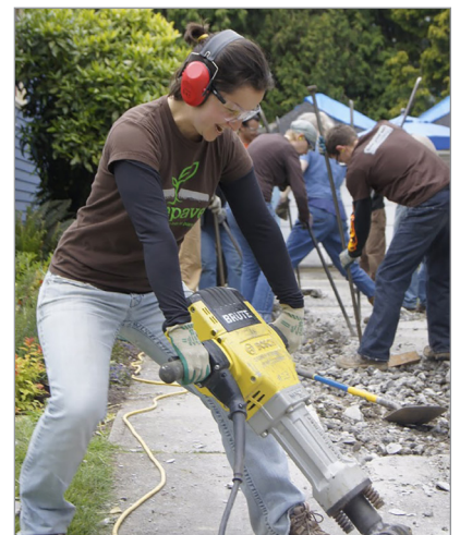
Jackhammer removing surfaces Photo credit: Eric Rosewall - Depave.org
