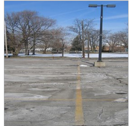
Parking lot with impervious area
