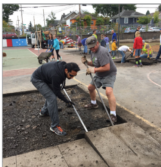
Volunteers removing section of concrete Photo credit: Eric Rosewall - Depave.org
