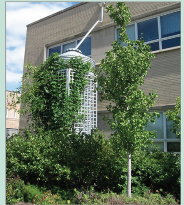
Cistern with lattice for decorative greening Photo credit: Abby Hall, EPA
