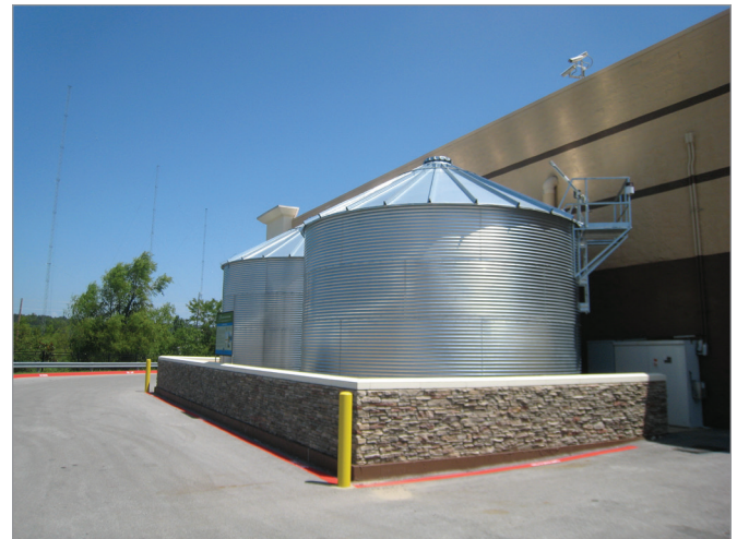
Walmart cistern, Fayetteville, AR
