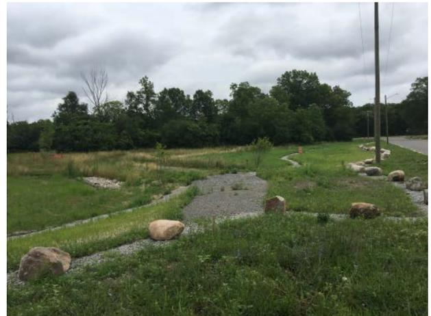
**Figure 10 Tireman Bioswales – Drainage Areas**
